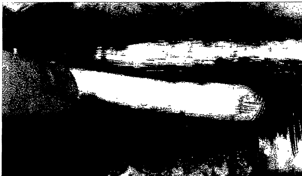
a) Level 1 fire damage — Surface charring only
