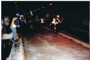
Sufficient curing must be provided to prevent shrinkage cracks
