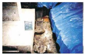
Exposing reinforcement bars at the head of newly constructed piles
