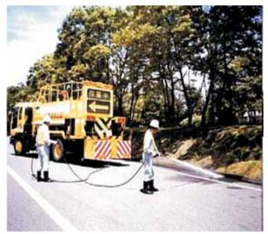
Fig. 6.05H Jet Water Cleaning
