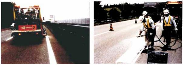
Fig. 6.05L Road Marking Equipment
