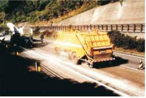
Tack coat is applied after sweeping and cleaning to enhance the adhesion between the new asphalt mixture and the existing pavement surface. Additional care shall be taken in applying tack coat on the milled vertical face.
