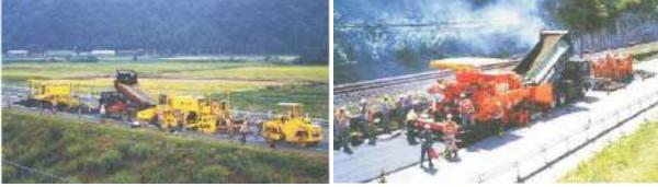
Typical fleet of equipment for in-situ recycling
