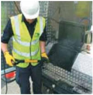
Step 4 : A small amount of material from the on-board 'hot box' in the vehicle may be added as required. Because the existing material is rejuvenated and reused, the amount of new material needed is minimised. The area is then raked and compacted by a portable plate vibrator transported in the vehicle to create a seamless joint.
