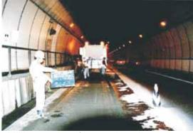
Milling road surface and loading scraps
