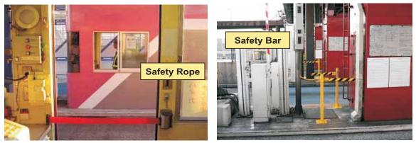
Fig. 1.14 Typical Safety Rope and Bar
