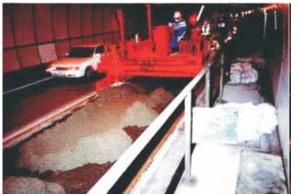
Concrete is generally placed mechanically to a thickness of 40 to 50 mm
