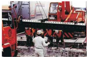
Installation of new joints and bar arrangement Reinforcing bars are placed for tight connection as required
