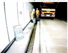
Cleaning of Drains with Hot Water Jet
