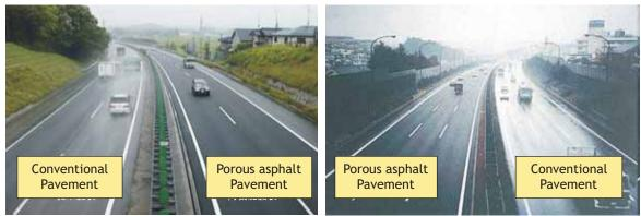
Fig. 6.01 Typical Porous Asphalt on Expressway
