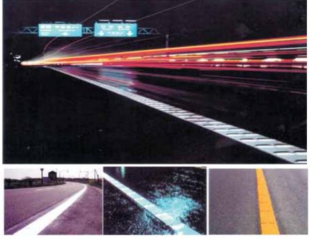
Fig. 6.03 Typical Road Markings for Improved Day/Night Visibility
