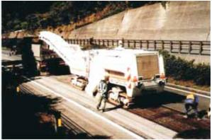
Milling the road surface and loading scraps
