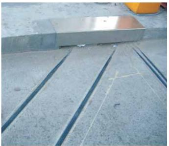
Fig. 1.04 Piezo Electric Sensors and Inductive Loops
