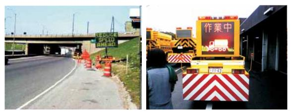
Fig. 2.08 Portable VMS in Operation in a Work Zone (Source: FHWA Manual and Japan Document)
