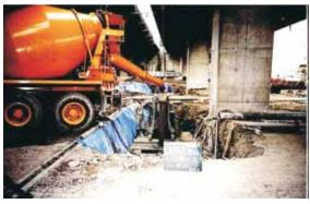
Concrete casting of new piles in progress
