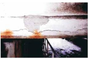
Concrete Cracks by Corrosion
