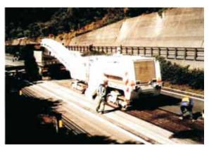
Fig. 6.05J Milling and Recycling Machine
