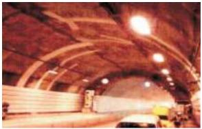
Treatment of Sprayed Concrete Fig. 6.04 Typical Repair Arrangement on Leakage Area
