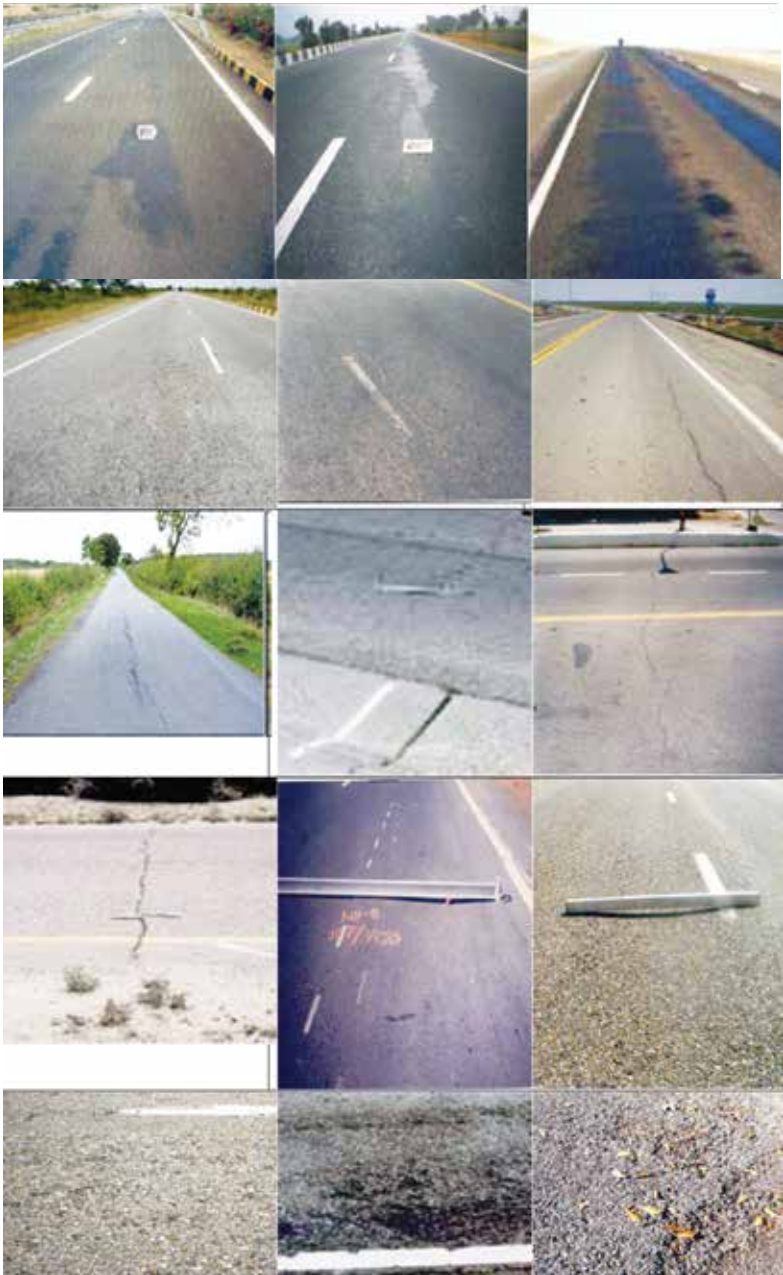
Annexe 12.1. Photographs of Distress on Flexible Pavements
