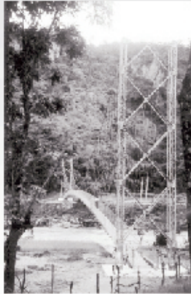
Khenjya Ghat bridge Baglung
