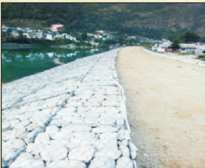
Fig 20 a & b : Photograph of Gabion mattress for slope protection on River & Road
