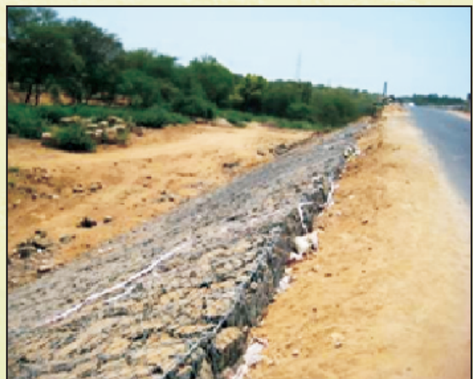
Fig 20 a & b : Photograph of Gabion mattress for slope protection on River & Road
