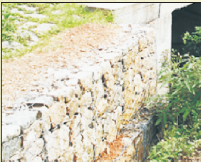
Fig 9: Typical photos of Gabion wall for along the road side
