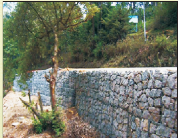
Fig 27a&b : Gabion Retaining wall for Road stabilisation in Rural Roads
