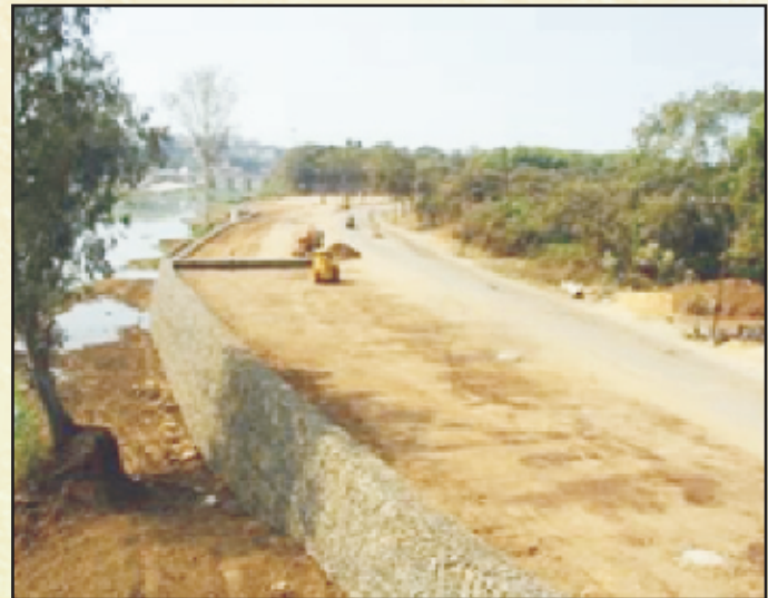
Fig. 26a&b: Gabion wall for Earth retention at Road side
