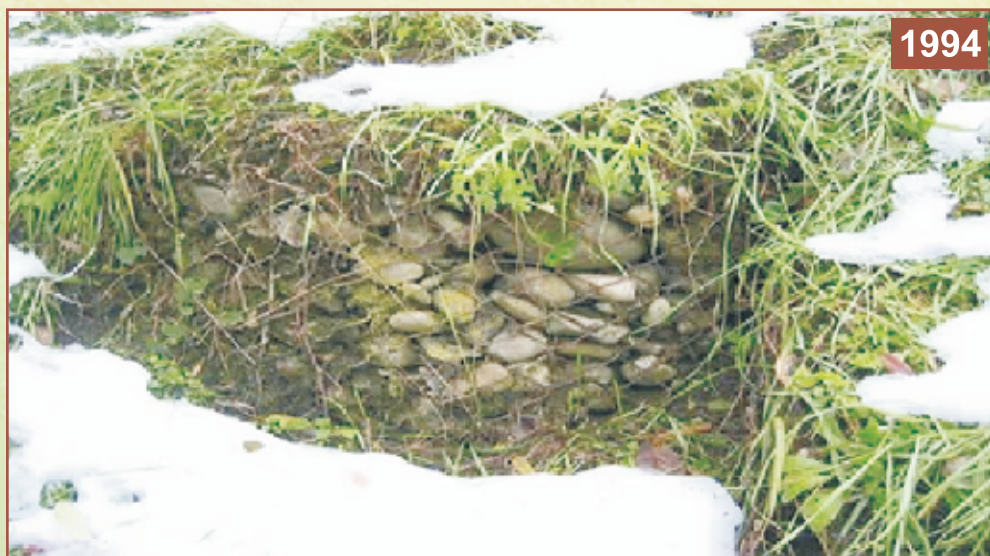
Fig 1a, b & c: Photograph depicts mechanical woven Gabions to protect Reno river bank
