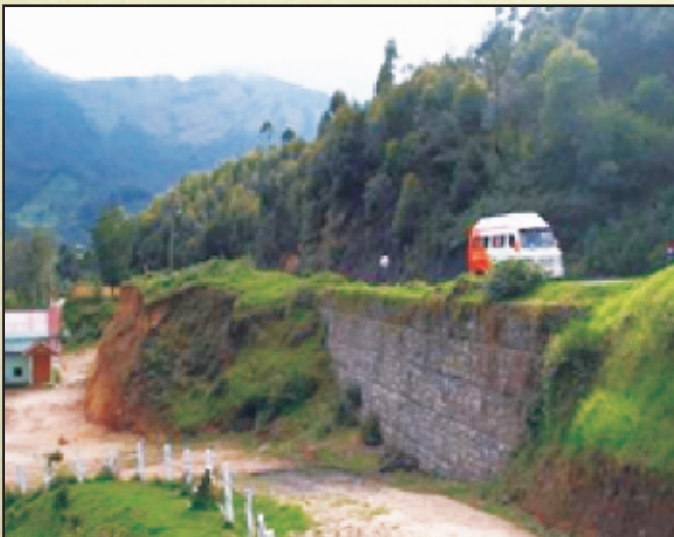
Fig 27a&b : Gabion Retaining wall for Road stabilisation in Rural Roads
