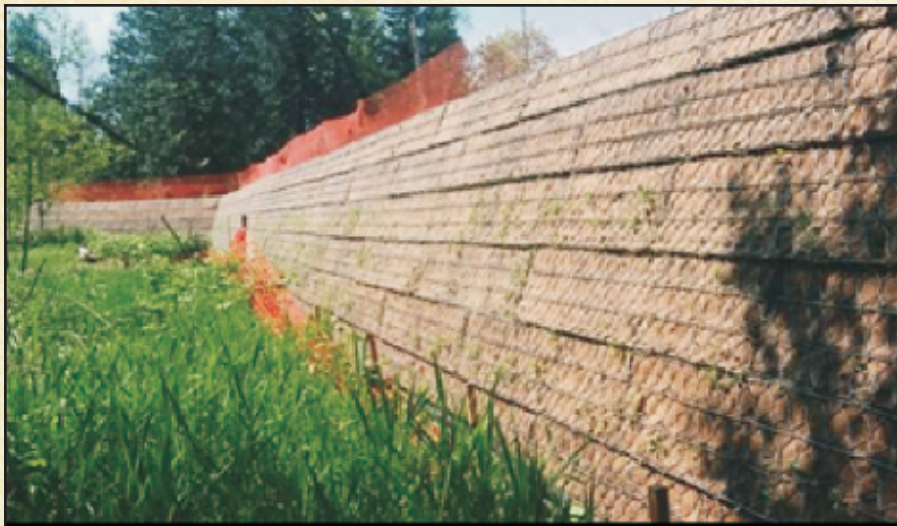
Fig 31 : Soil reinforced slope with Green facia at road side
