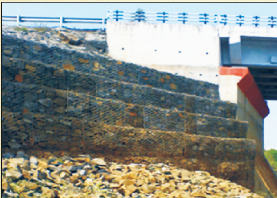
Fig 17: Photograph of Minor bridge protection with Gabion retaining wall
