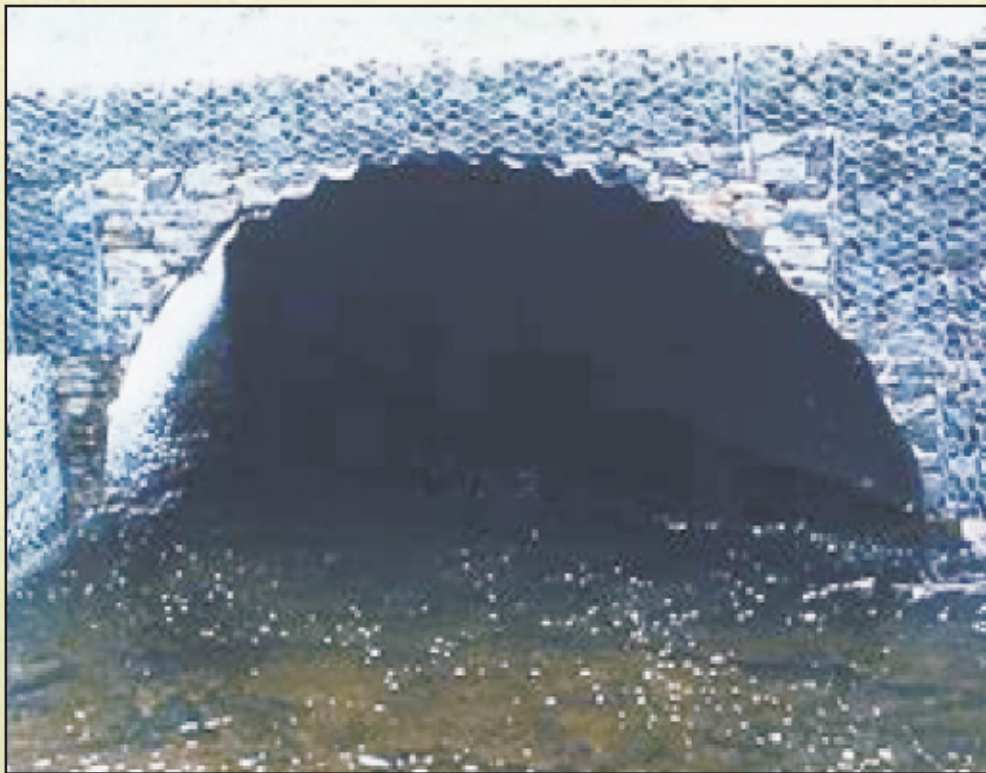
Fig 13: Typical Photo of Culvert with Gabion Gravity Retaining wall
