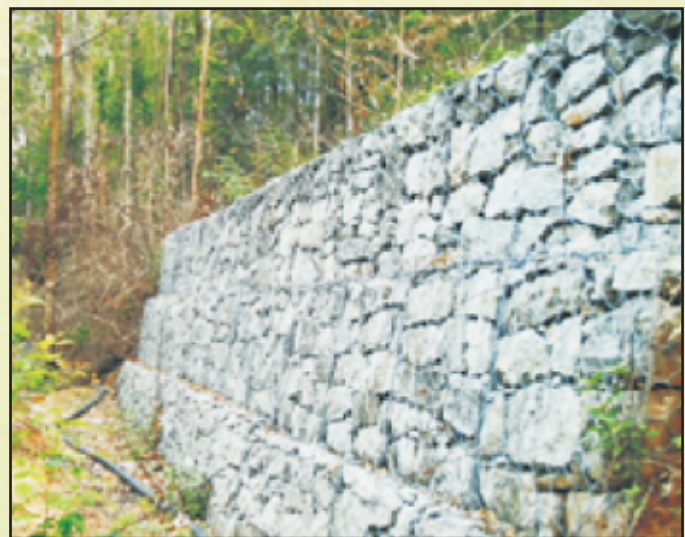
Fig 9: Typical photos of Gabion wall for along the road side
