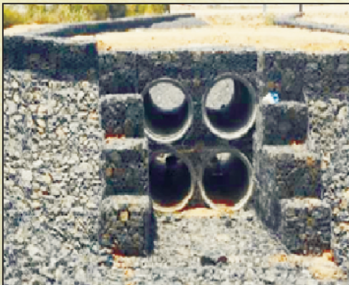
Fig 15a,b&c : Photos of multiple pipe protection with Gabion Gravity Retaining wall
