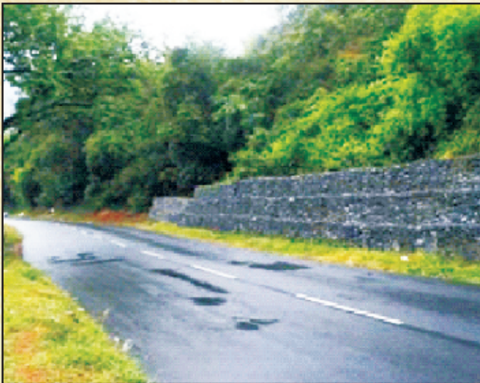
Fig. 26a&b: Gabion wall for Earth retention at Road side
