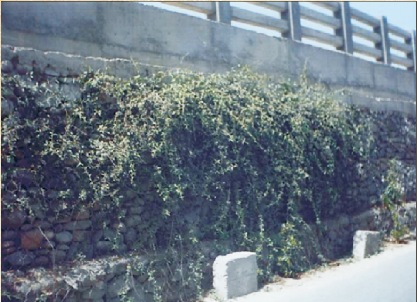
Fig 29 : Typical photo of Reinforced soil wall with Gabion facia
