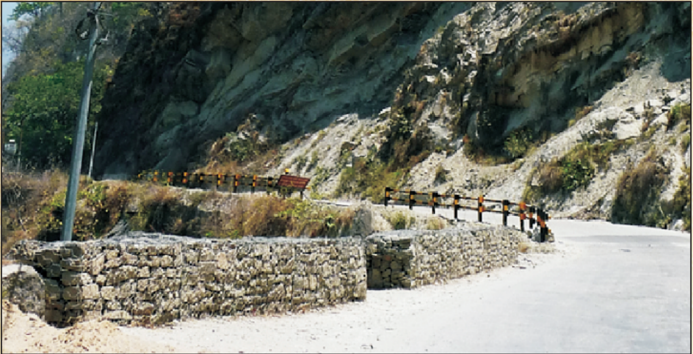
Fig 23 : Photo depicts Gabion wall as crash Barrier on Sharp Curve on Hilly Road
