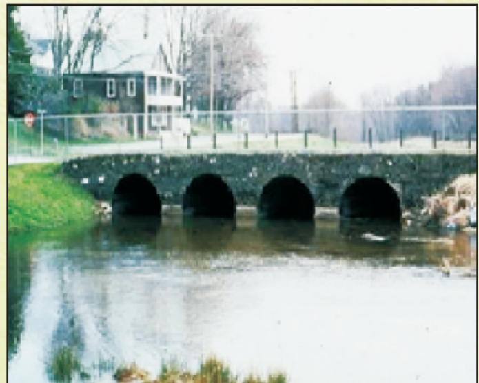
Fig 15a,b&c : Photos of multiple pipe protection with Gabion Gravity Retaining wall
