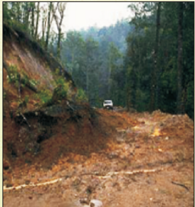
Fig 24 a & b: Typical Road Failure problem
