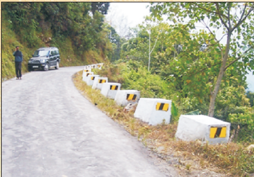
Fig 21 : Photo of Concrete crash Barrier on Sharp Curve on Hilly Terrain
