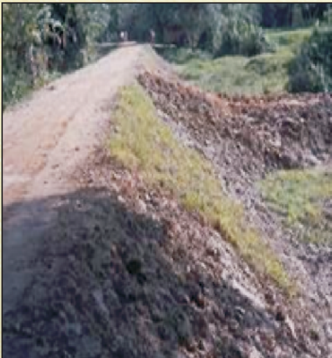
Fig 24 a & b: Typical Road Failure problem
