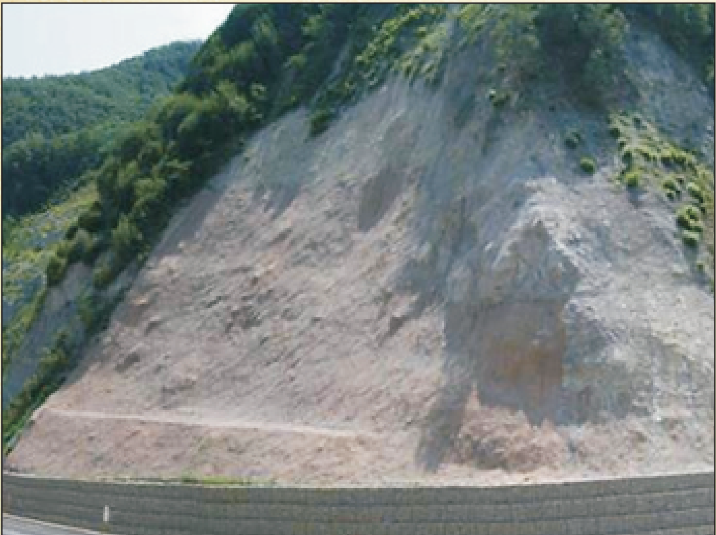
Fig.33: Photos depict Gabion toe wall on Valley side of Road
