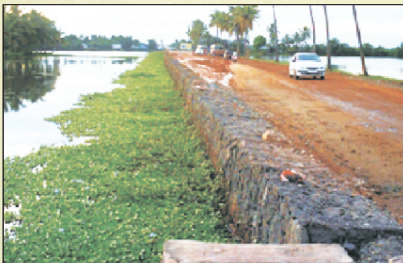
Fig 11a,b &c : Typical photos of river bank protection with Gabion wall along road
