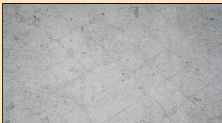
Figure 11 Appearance of Top Surface of Cell-Filled Pavement
