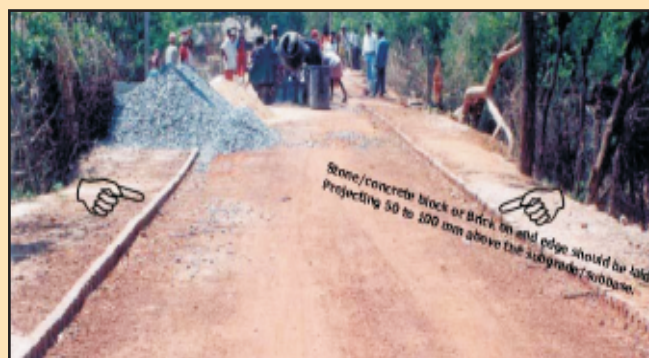
Figure 6 Stone/concrete block of Brick on end edge
