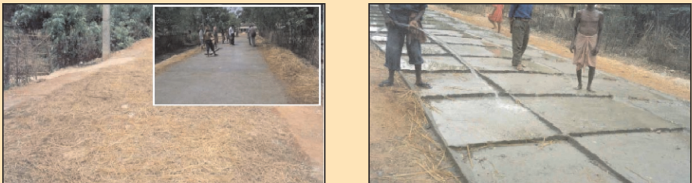
Figure 10 Curing of concrete by wet paddy straw and ponding
