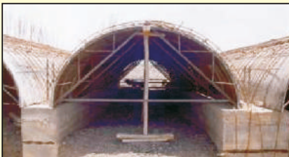
Cement Concrete Block Arches in place of Hume Pipe
