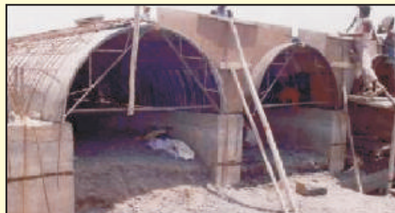
Cement Concrete Block Arches in place of Hume Pipe
