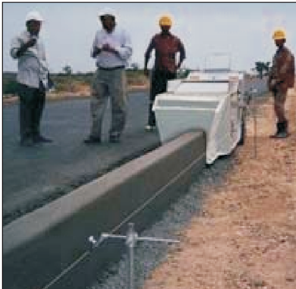
Fig. 10.24 Kerb Laying Machine
