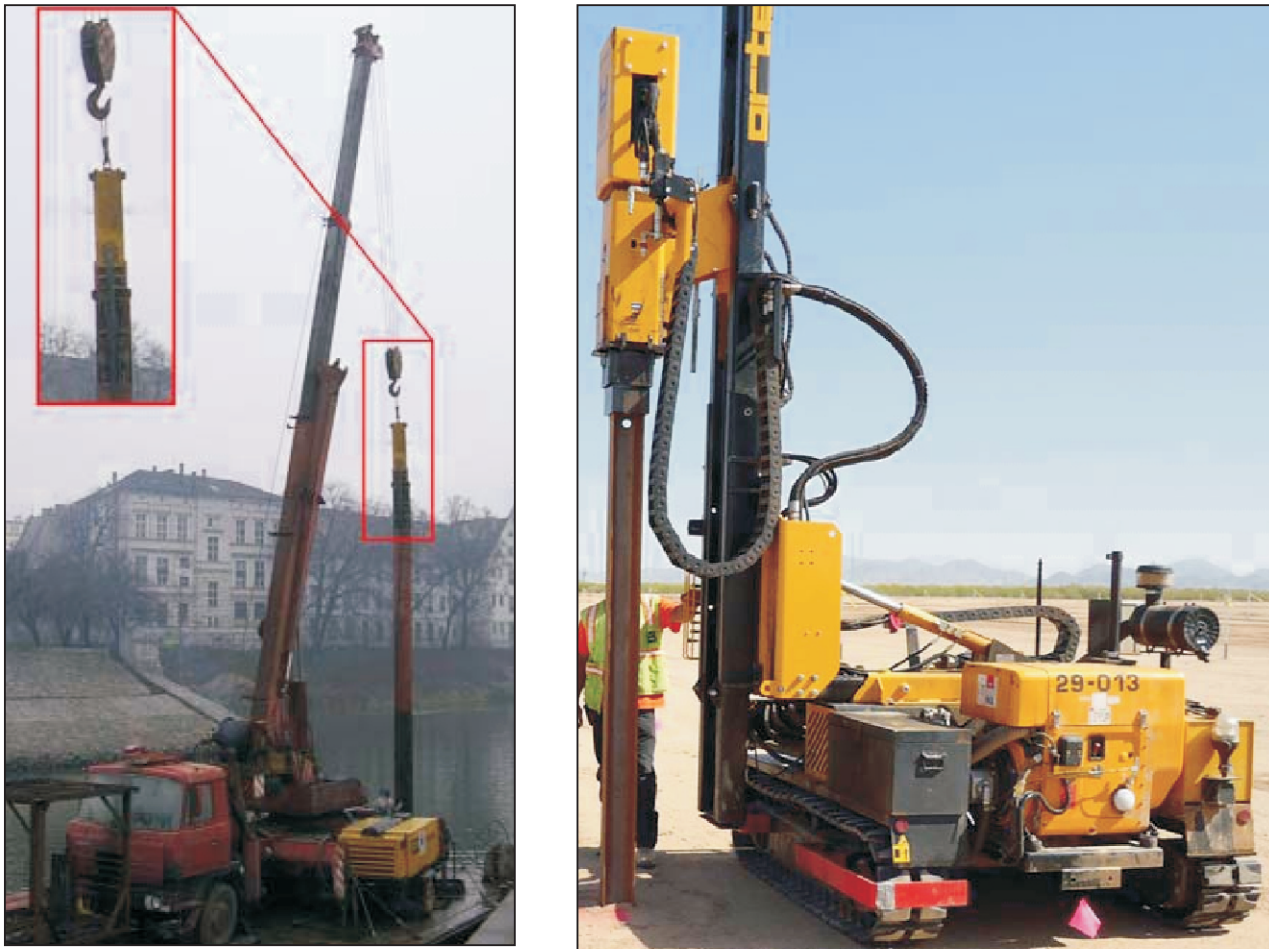
Fig. 13.2 Pile Driving Equipment in Operation
