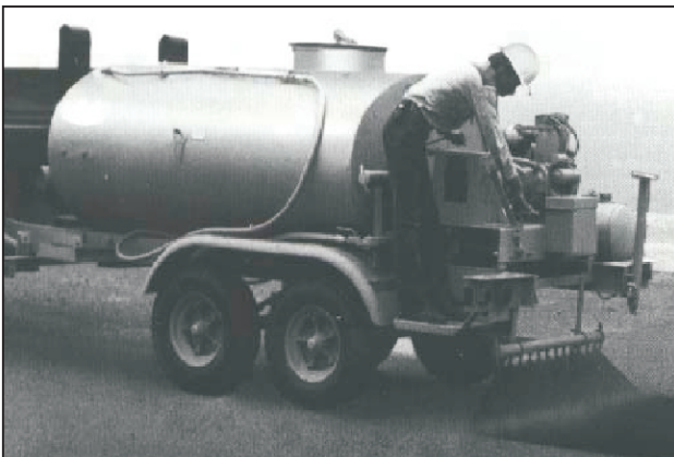
Fig. 9.2 Spray Bar in Operation in Tractor Towed Bitumen Pressure Distributor
