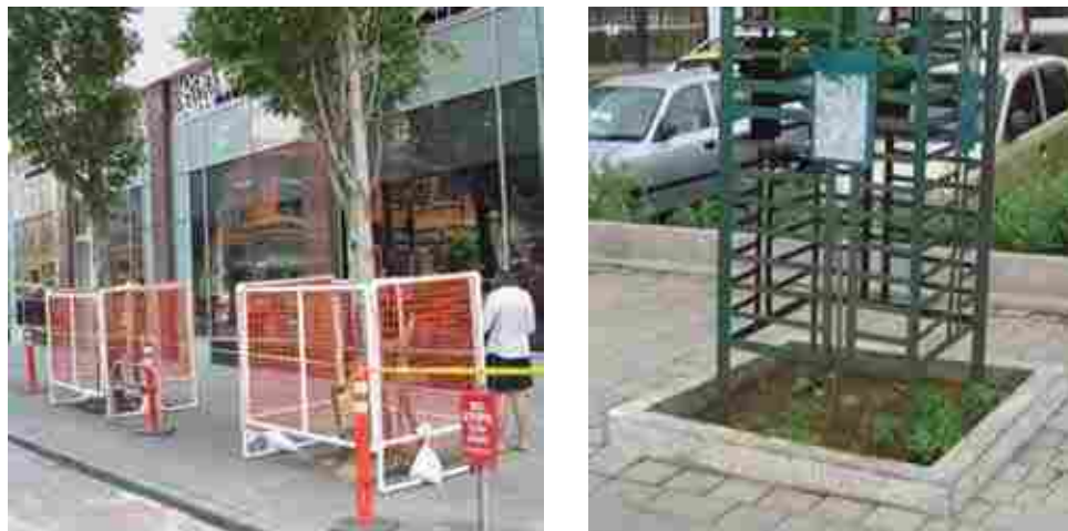
Fig. 103 Installation of Tree Protection. Right: Example of Tree-pit with Skirting Around – acts as an Impediment for Pedestrians, prevents Rainwater from reaching the Roots and is not advisable
