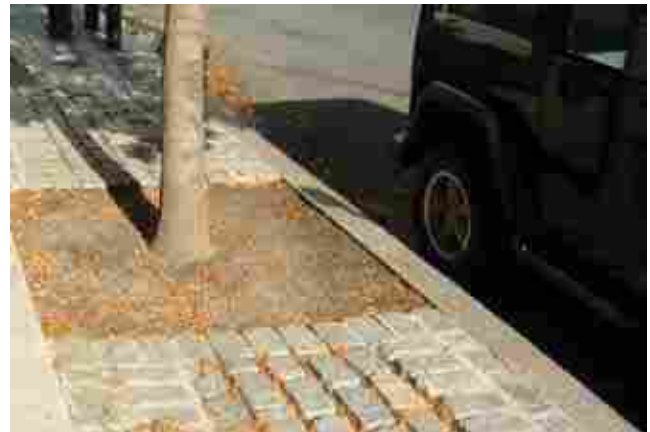
Fig. 95 Tree-pit Detail without Seating (note: unplanted tree-pits are not recommended)
