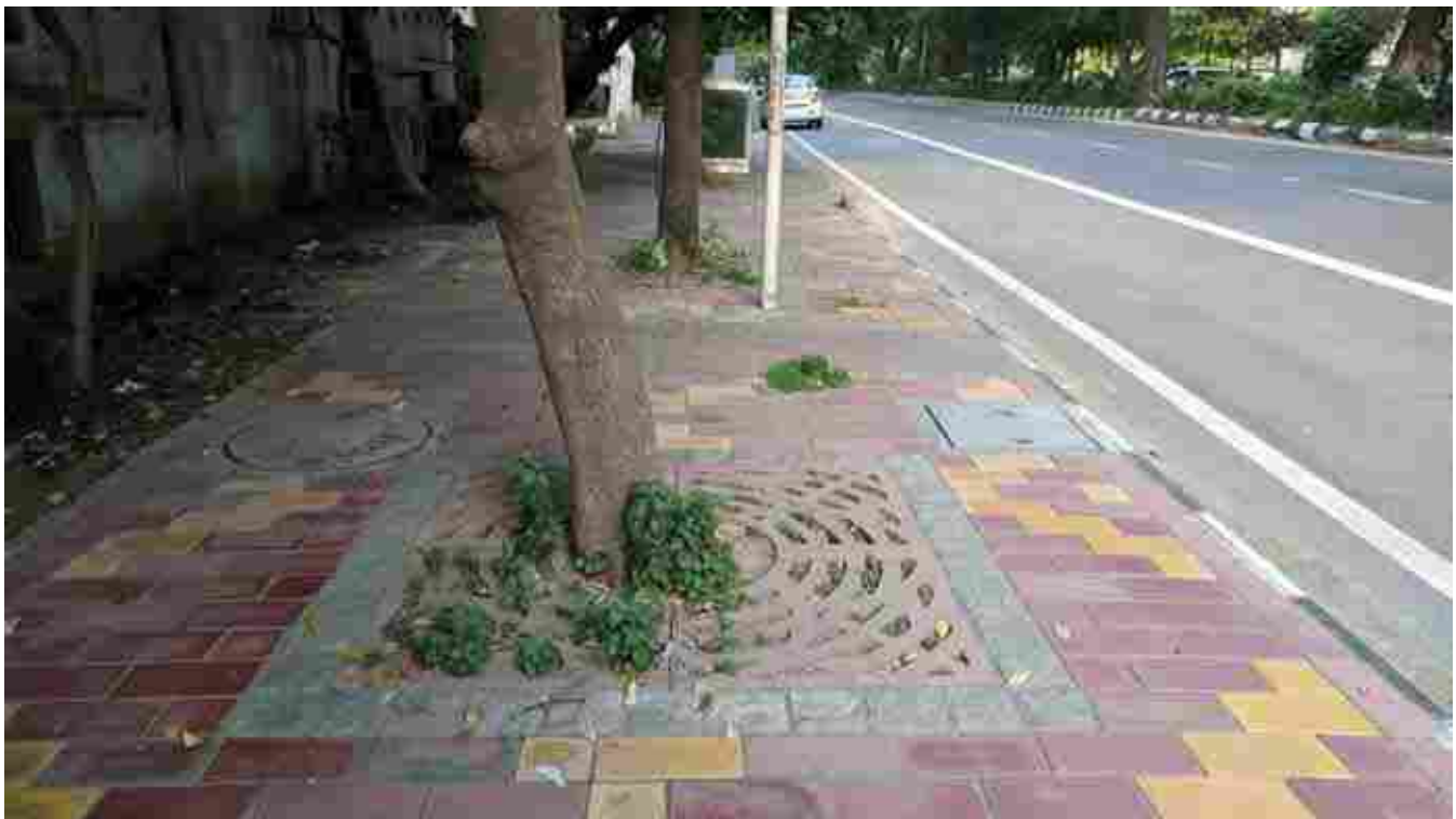
Fig. 107 Tree Grating that allows Water to seep through and Plants to peep through, while allowing People to Walk Over
