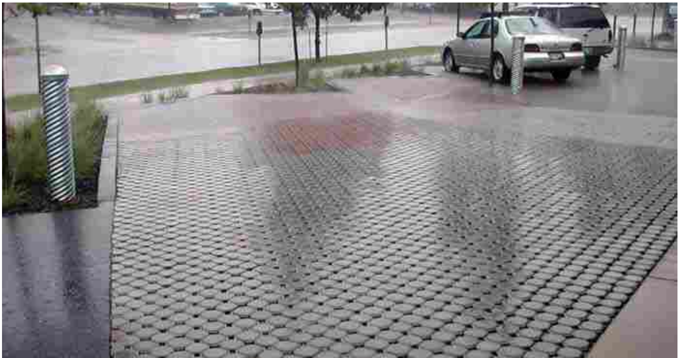
Fig. 46 Example of Permeable Paving used within the Parking Area within MFZ
