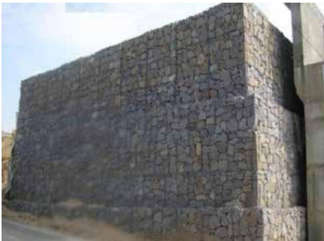
**Fig. 1a Soil Retaining behind an Abutment**
