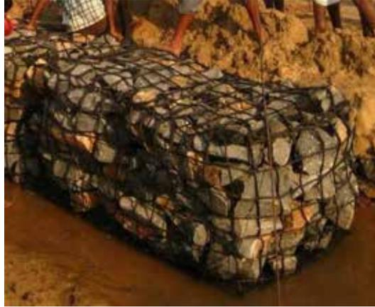
**Fig. 3: Polymer Rope Gabions**
