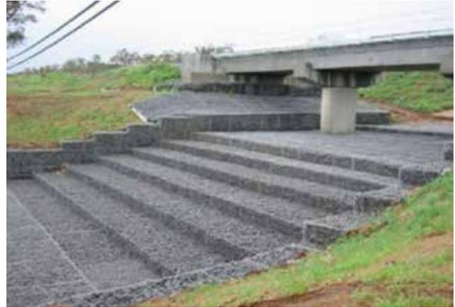
**Fig. 1d Bridge Abutment Protection**
