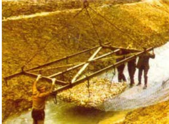
**Fig. 38: Underwater placement of Revet Mattress by Crane**
