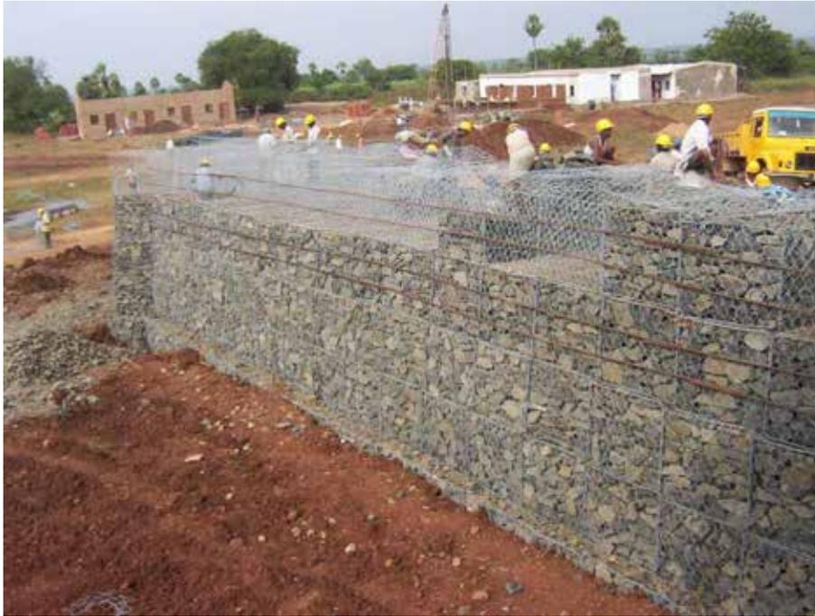
**Fig. 35: Lid closing Procedure at Site**
