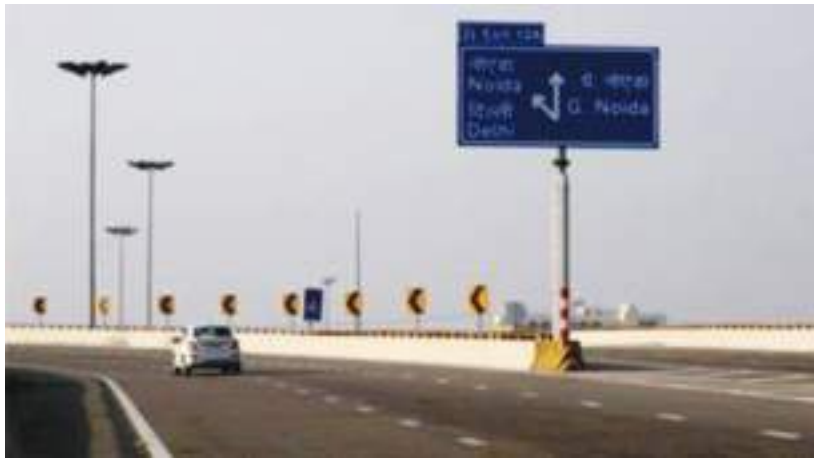
Fixed hazards in gore areas on high speed roads are especially hazardous
