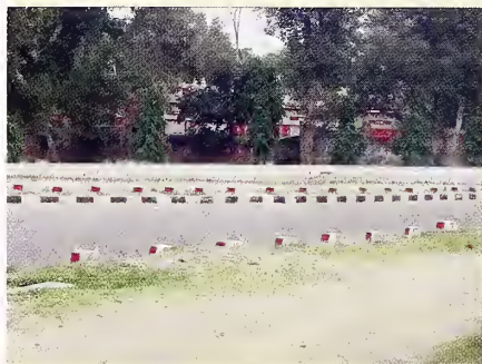
Reflecting Kerbs for Night-time Visibility on Curves
