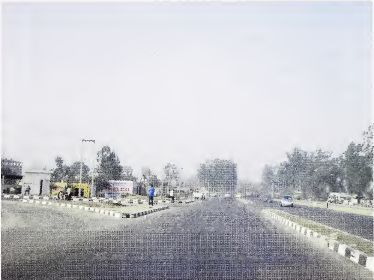
Fig. 5.16 Large Channelising Island
