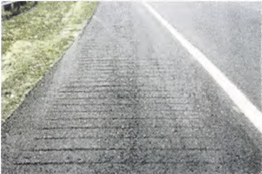
Fig. 5.22 Rumble strips on Shoulder to Alert Drivers who have Strayed from Carriageway before Sharp Curve
