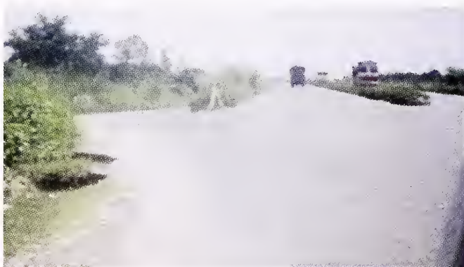
Fig. 5.17 Lack of Details at Access Points and Minor Junctions Fail to give Proper Guidance to Motorists
