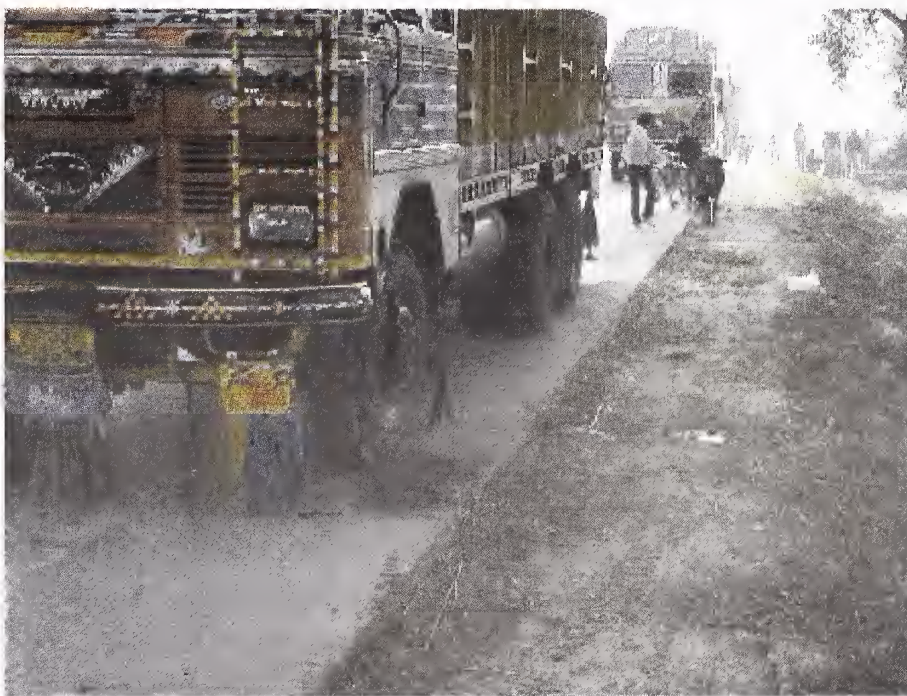
Photograph 1 - Erosion, Wear and Tear of Soft Earthen Shoulder. Trucks Preferring to Park on Outer Lane
