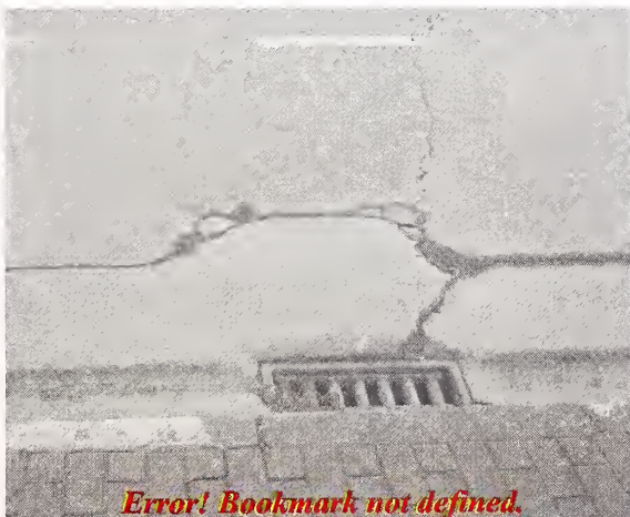
Photo 11) Manhole / Inlet Cracking Failure
