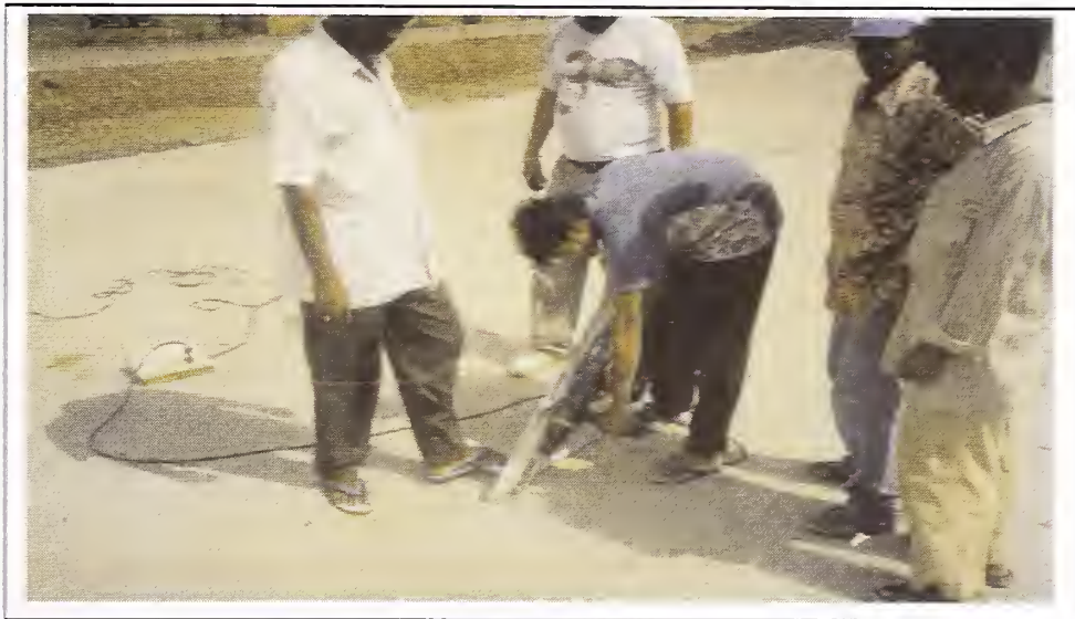
Fig. 7.2. Drilling the Inclined Holes with Angle Template
