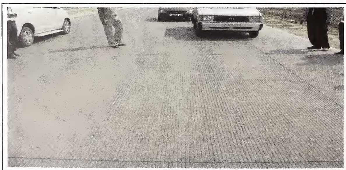
Fig. 8.7. Abrasion in the Wheel Paths (Longitudinal Tining)
