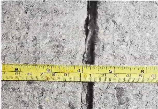
a) The Liquid Sealant Adhesion Failure
