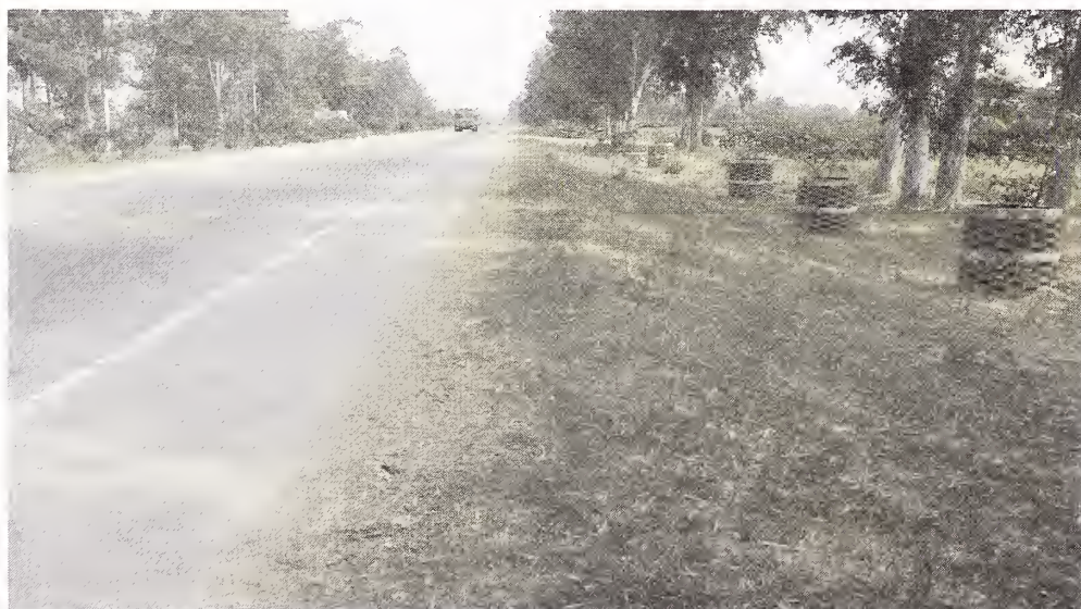
Photograph 3 - Turfing on Shoulder and Side Slope
