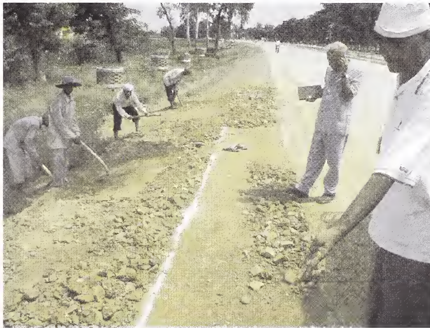
Photograph 4 - Construction of Hard Shoulder with Recycled Sub-Base/Base Material Recovered from Existing Highway Mixed with Local Red Moorum (CBR>30)
