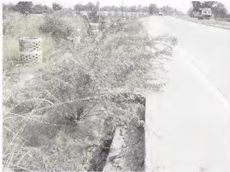
Photograph 2 - Complete Erosion and Undermining of Rigid Pavement has Commenced
