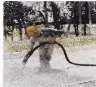
c) Compressed Air used to clean
