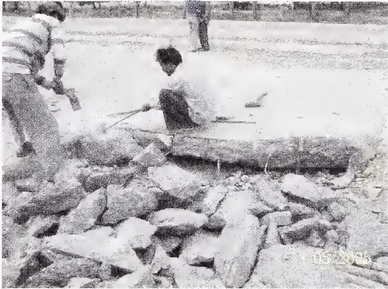
Photo 22) Shattered Slabs
