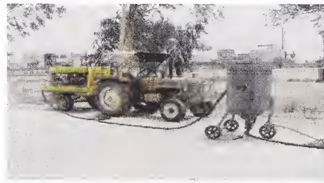
b) Sand blasting the groove after raking out the sealant residue and rubbish from the joint.
