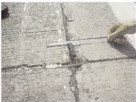
Photo 23) Compressive Seal - Loosening
