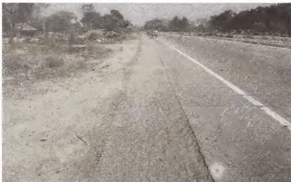
Photograph 5 - Construction of Brick on Edge (Paved Shoulder)
