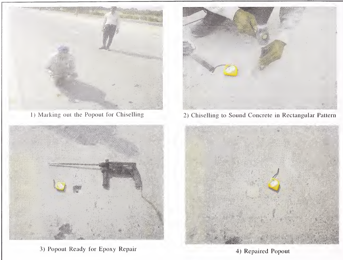
Fig. 8.5. Photographs Illustrating Repair of Popouts
