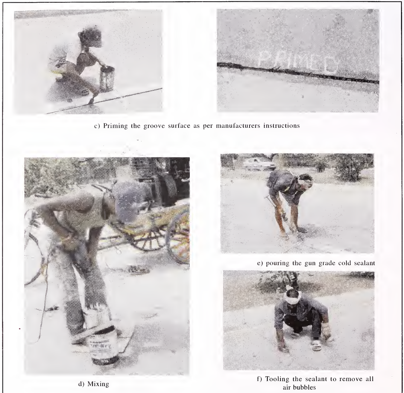
Fig 6.6. Priming and Reinstallation of PQC Joint Sealant
