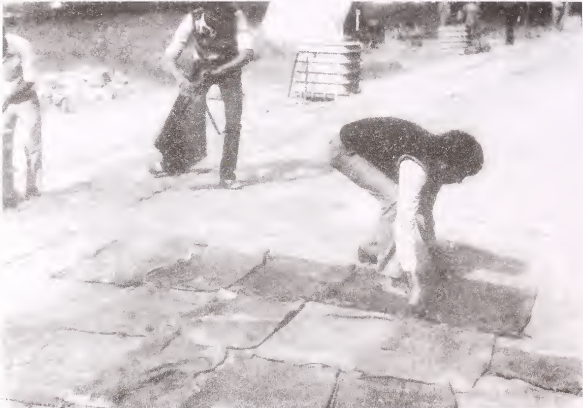
Fig. 3.9 : Curing by Covering the Compacted Stabilized Soil Surface with Wet Gunny Bags
