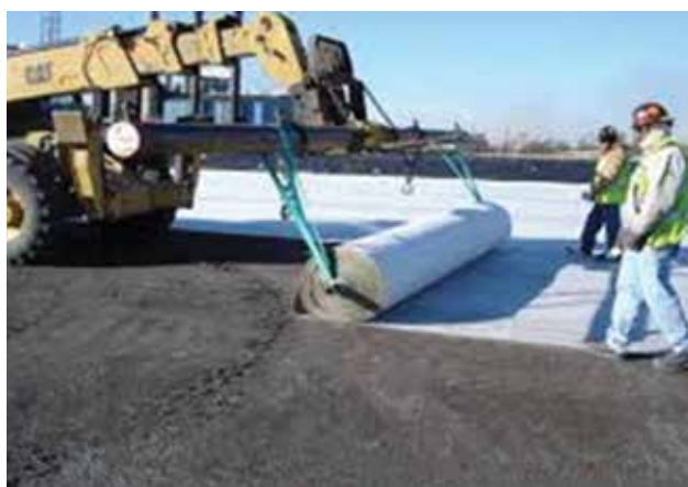
Fig. 6.2 Unrolling of Geosynthetic Roll
