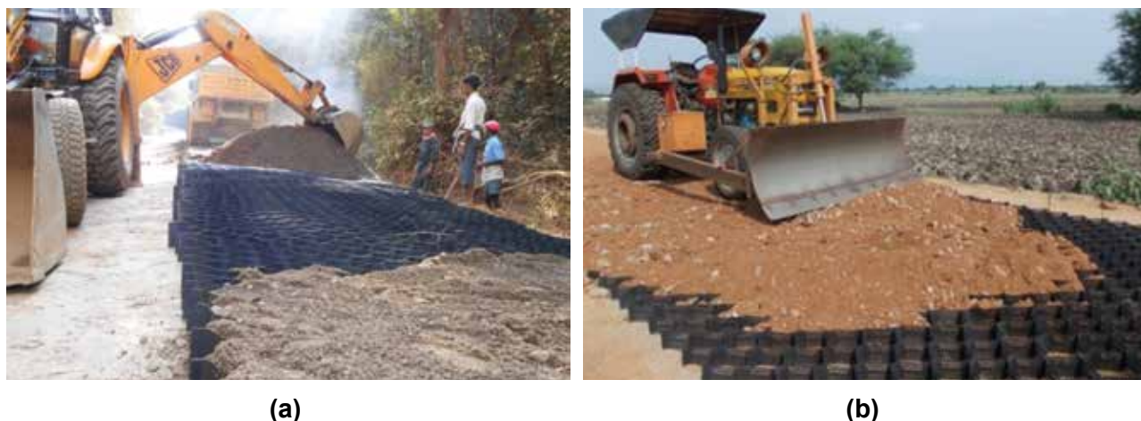
Fig. 6.6 (a) In Filling from Side, (b) Equipment Run on Geocell Filled with Soil
