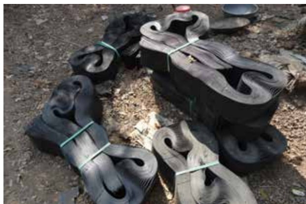
Fig. 6.3a Geocell Panels at Site
