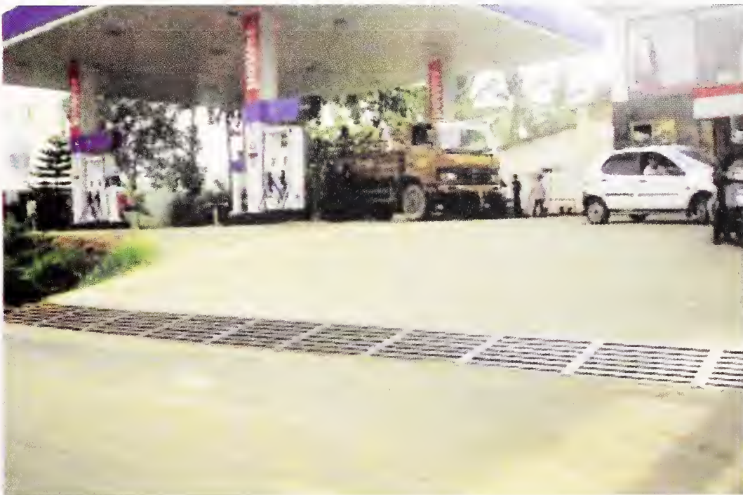
Photo. 9.5 (b) Showing Grating Provided at a MS/HSD Gas Outlet for Effective Discharge of Storm Water
