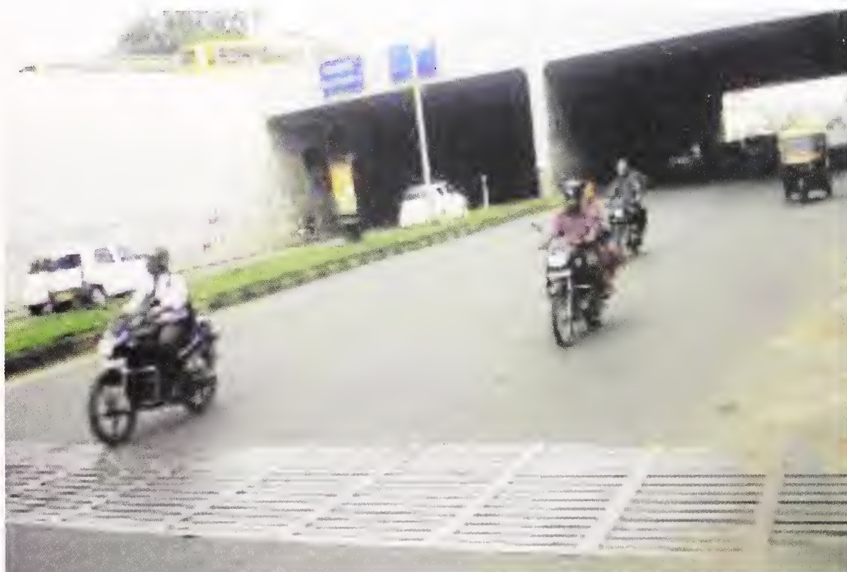
Photo 9.3 (a) Drainage of Subway by providing a Grating Across the Full Width
