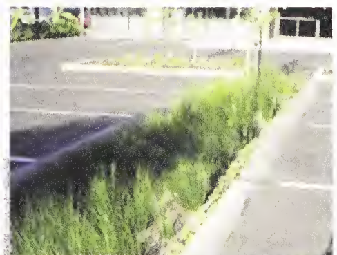
A stormwater planter within the interior median of a parking lot.
