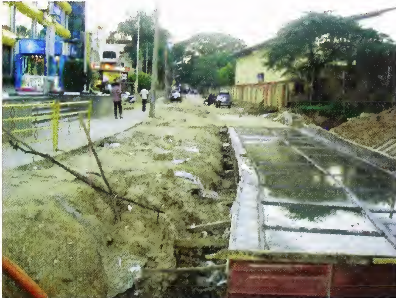
Photo 5.2 Box Drain in the Carriageway Portion of Road
