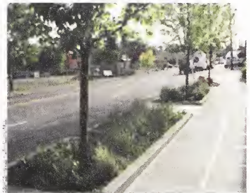
This arterial street was retrofitted with a series of stormwater infiltration planters.
