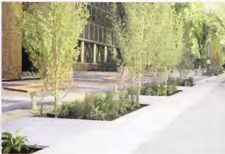
This green street features a continuous flow-through stormwater planter with multiple bridge pedestrian crossings
