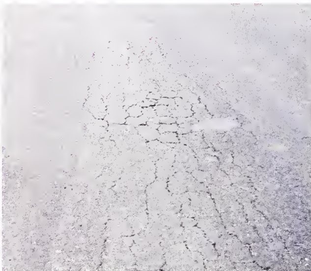
Photo 5.1 A Cracked and Settled Bituminous Pavement which Permits Seepage of Water
