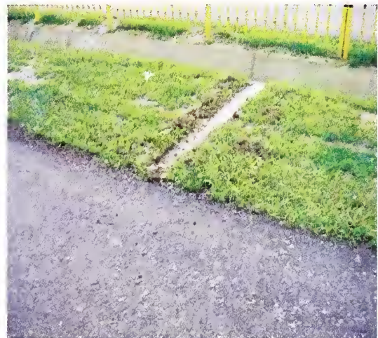
Photo 4.16 Naturally Grown Turf on Earthen Shoulder Causing Resistance to Disposal of Surface Water
