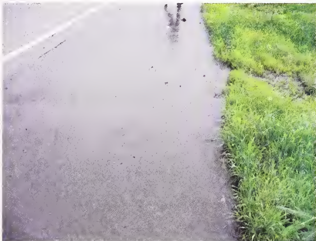
Photo 4.15 A View of Tall Grass Obstructing Surface Drainage
