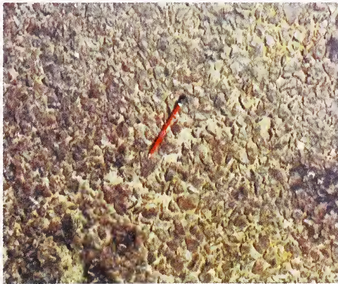
Photo 4.2 Texture of a Bituminous Pavement
