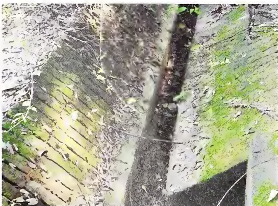
Photo 8.2 A Brick Lined Drain Provided with Smaller Secondary Channel
