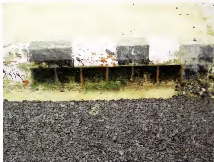
Photo 4.7 Steel Gratings Provided in CC Kerb as an Inlet
