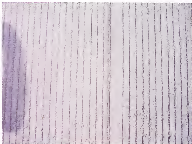
Photo 4.4 Tine Textured Concrete Pavement
