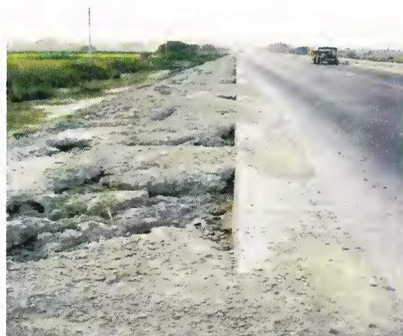
Photo 4.10 Severely Eroded Earthen Shoulder of Concrete Road
