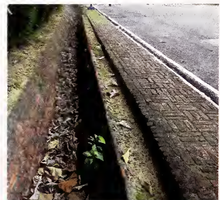
Photo 8.3 An Open Side-Drain with Brick Lining
