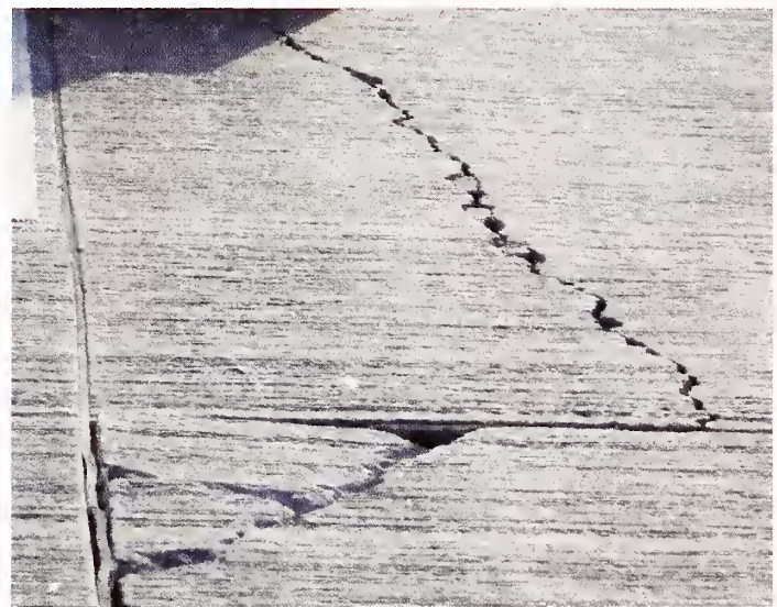
Photo 5.2 A View of a Cracked Concrete Slab which Facilitates Seepage of Water
