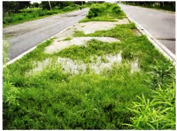
Photo 4.20 A Raised Median with Pool of Water which Eventually Seeps to Foundation Layers of Pavement
