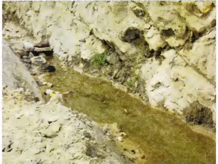
Photo 5.7 Stagnated Seepage Water in a Cut Section in a Hilly Terrain
