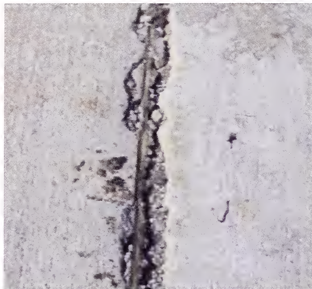
Photo 4.3 A Damaged Joint Groove can Permit Seepage of Water to Lower Layers
