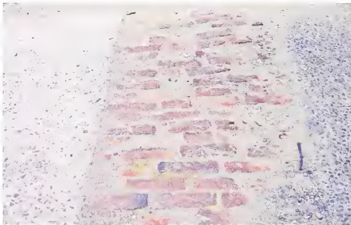
Photo 4.13 Brick Surfaced Shoulder
