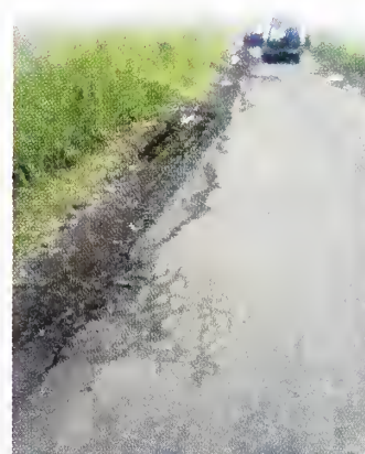
Photo 4.12 Earthen Shoulder of a Bituminous Pavement in Neglected Condition
