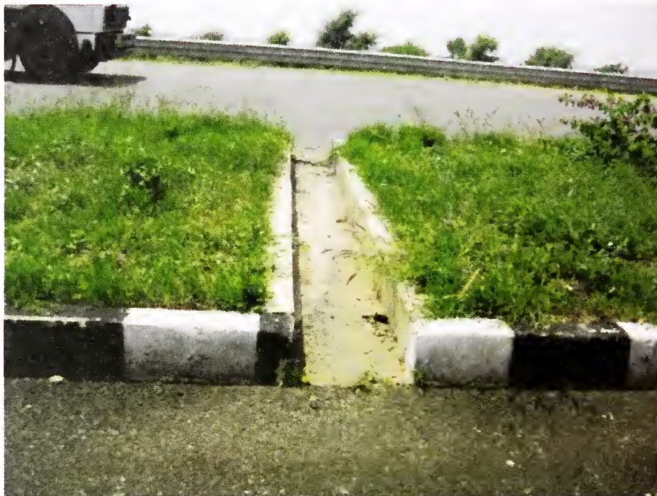
Photo 4.21 A Median Opening Provided in a Super Elevated Section for Draining from One Carriageway to Another
