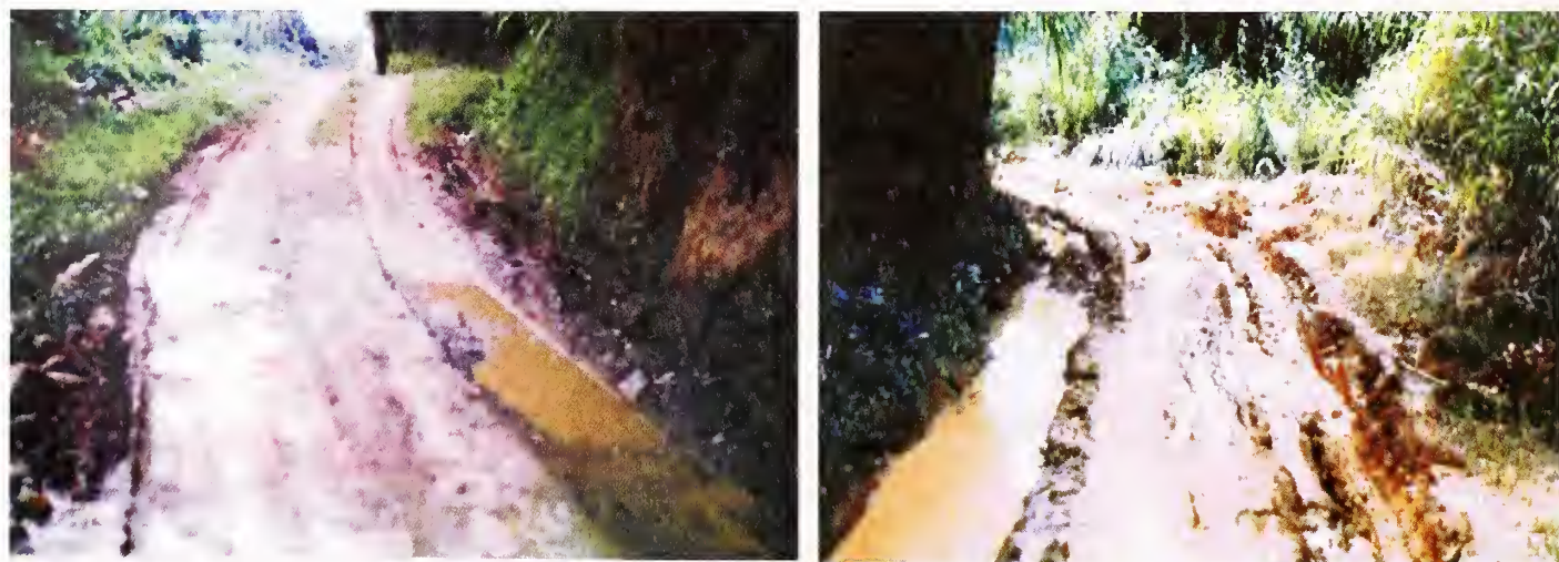
Fig. 8.15 Damage to Road Surface Due to Inadequate Drainage
