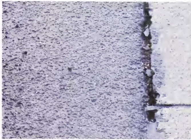
Photo 5.5 An Open Joint Between Concrete Pavement and Bituminous Shoulder
