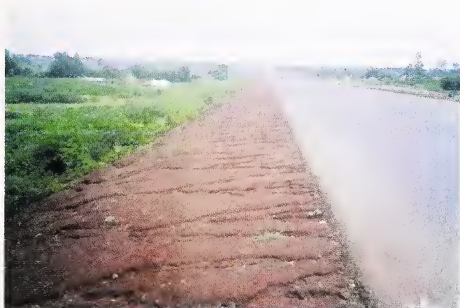
Photo 4.11 Limited Erosion Seen on a Shoulder Constructed with Granular Material
