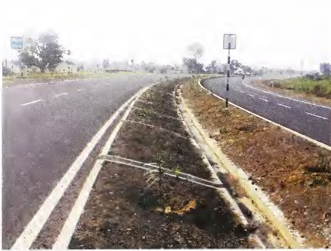
Photo 4.19 A Depressed Median with Lined Median Drain and Chutes
