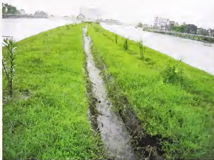
Photo 4.18 A View of Depressed Median with Lined Drain. Turfing as Grown Naturally on the Earthen Sections
