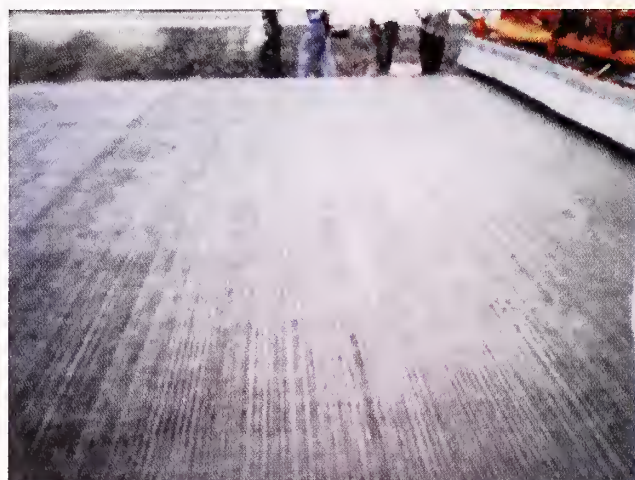
Photo 4.5 Brush Textured Concrete Surface
