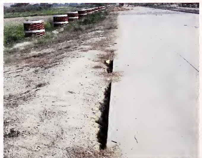
Photo 5.4 A Large Opening in Longitudinal Joint Between Concrete Pavement and Earthen Shoulder
