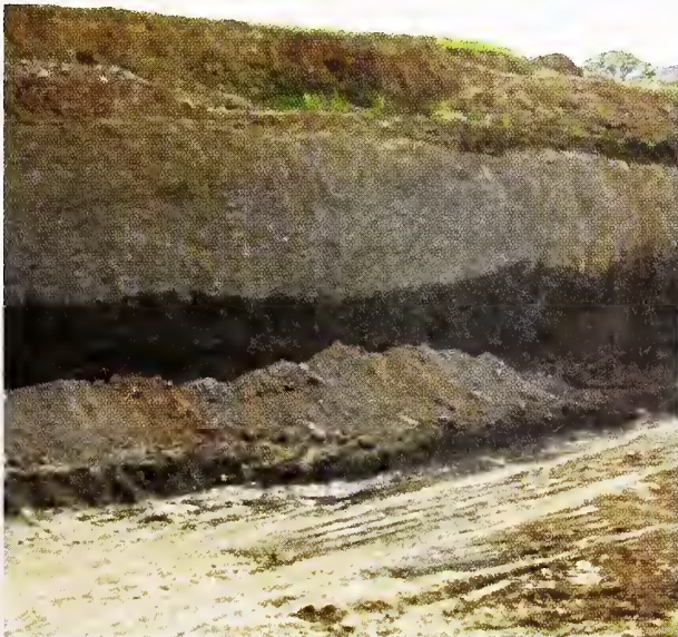
Photo 5.6 Seepage Taking Place through Soft Sandy Soft Rock
