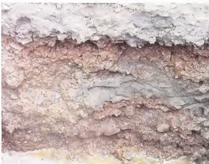
Photo 5.3 Subsurface Water Found at Subgrade Level in a Road
