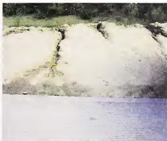
Photo 4.9 Eroded Earthen Shoulder of a Concrete Road
