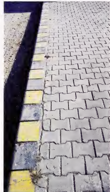
Photo 4.14 Shoulder Paved with Concrete Blocks
