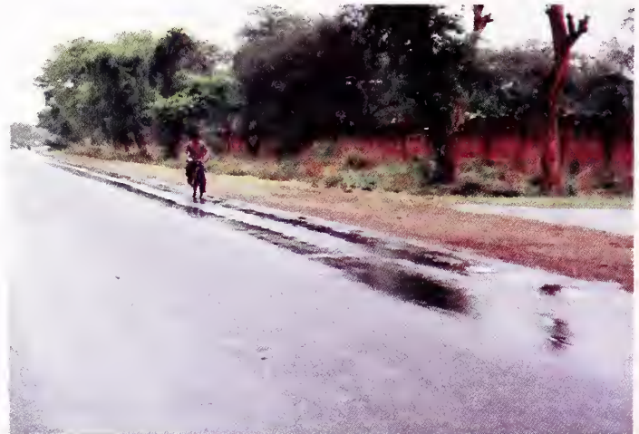
Photo 4.1 A Film of Surface Water which can Lead to Hydroplaning
