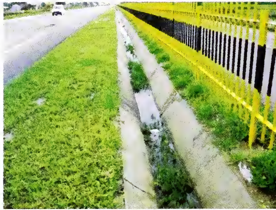
Photo 8.1 A View of Precast RCC Lined Drain
