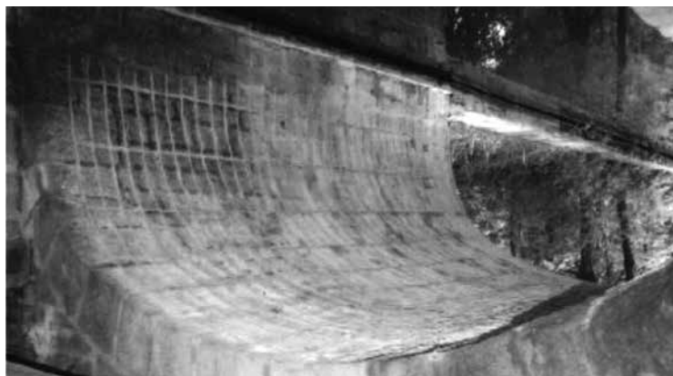
Fig. No. 5.1 (b) A Helical Reinforcement Provided in one of the Arch Bridges
