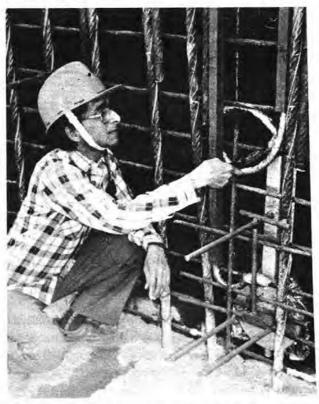
Fig. 3.29.1. Pressure Cell Assembly in Position before Concreting 169
