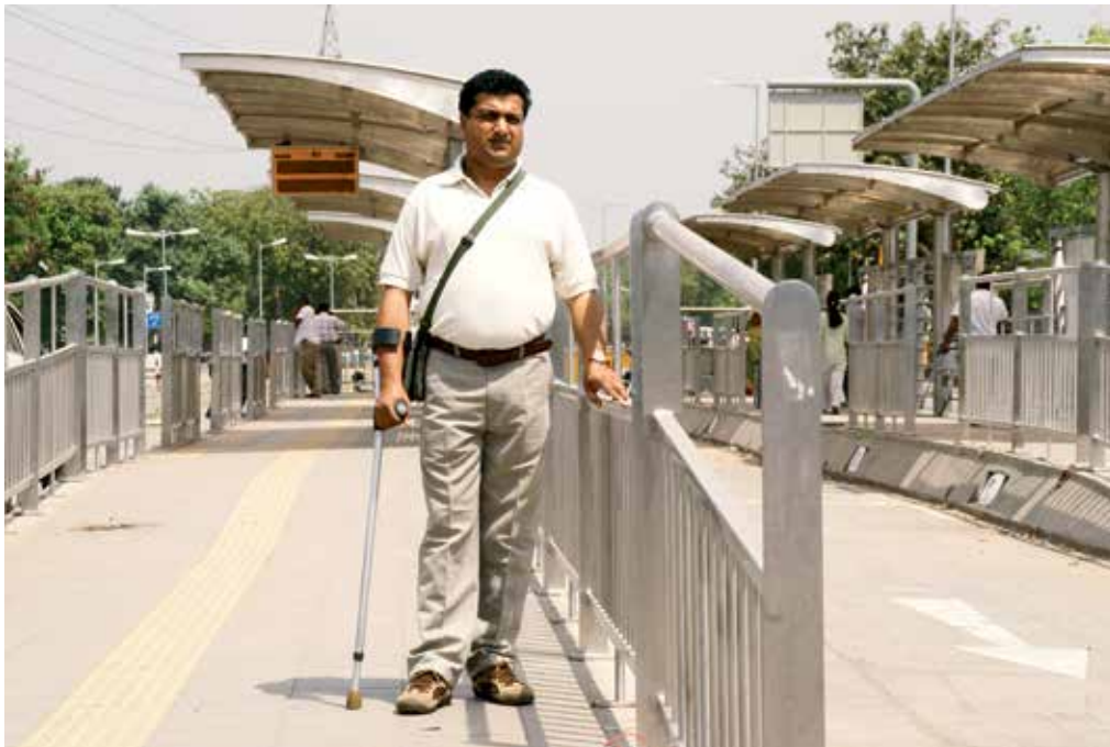
Photo 33: Ramps at stations should have a 1:15 gradient max. and handrails at two levels on both sides of the ramp (Photos courtesy(R) SAMARTHYAM)
