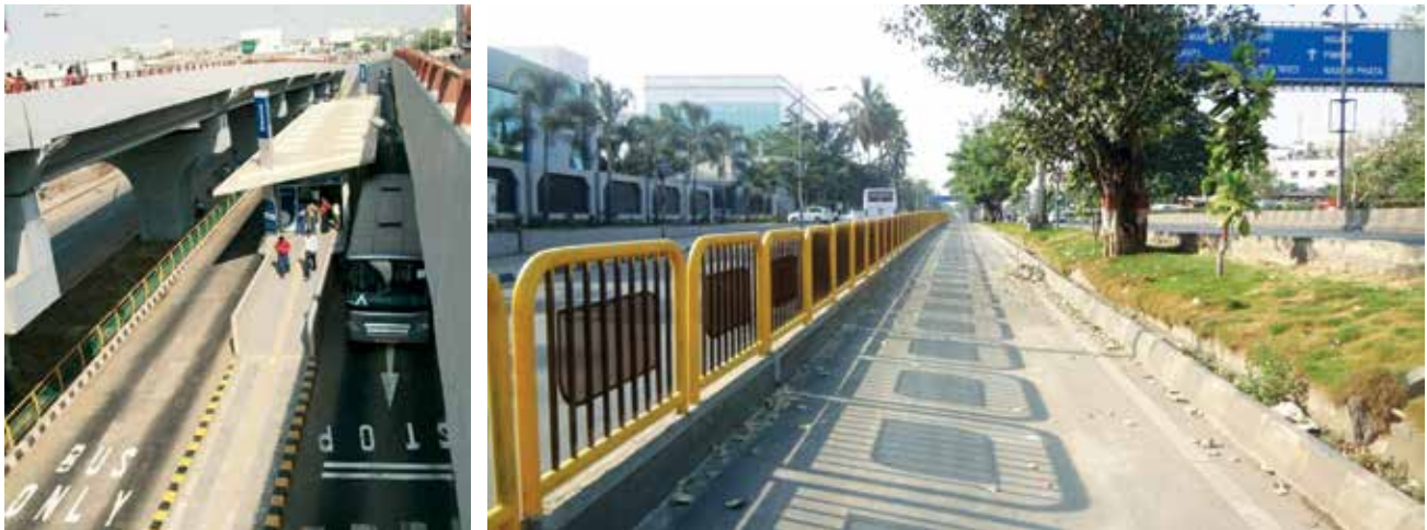
Photo 26: In Ahmedabad, a split flyover allows for continuous BRT movement in the median (left). In Pimpri Chinchwad, BRT lanes were constructed in the service lane in order to accommodate existing express lanes (right)
