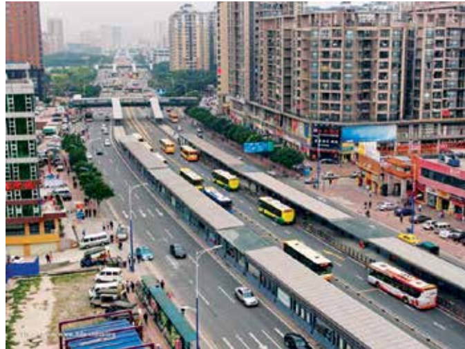
Photo 18: An average spacing of 300 to 800 m between stations is optimal for passengers.
