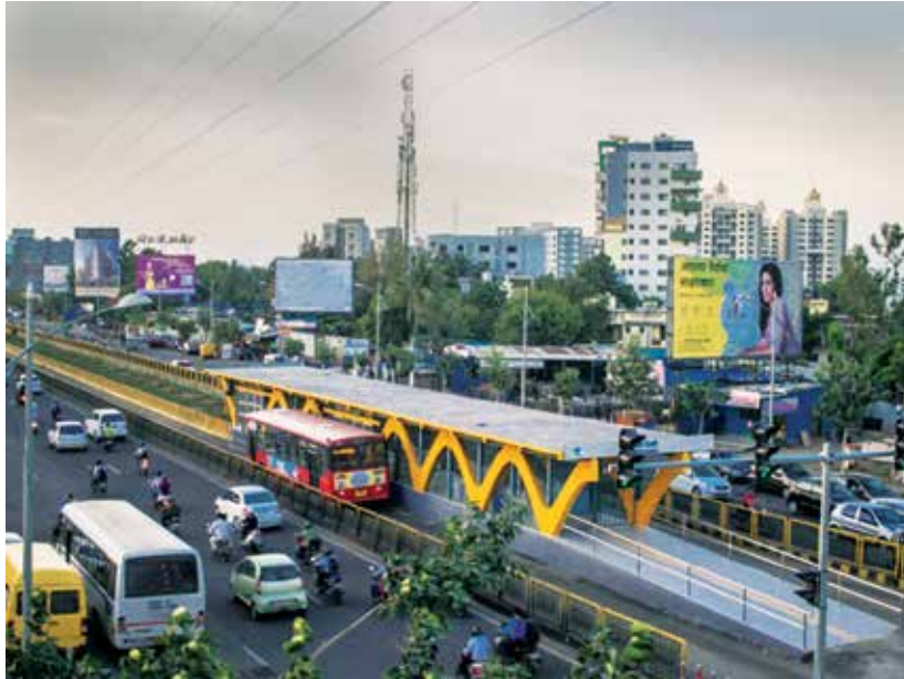
Photo 8: Median stations, such as in Pimpri Chinchwad are less expensive and have a more compact footprint than side stations.
