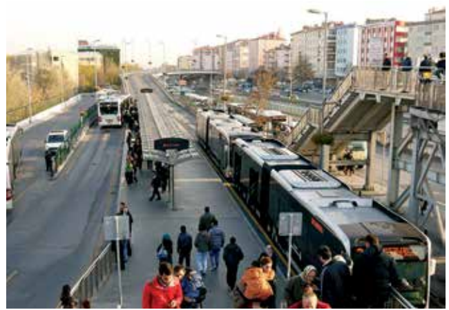
Photo 32: Safe at-grade pedestrian crossings, in Dar es Salaam (left), are preferred as they provide easy, convenient access to BRT stations. On highways corridor such as in Istanbul (right), foot overbridges can be considered
