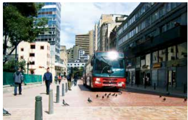
Photo 27: Quito BRT utilises reinforced concrete to ensure the longevity of BRT lanes (left). For aesthetic reasons, Bogota utilises brick and paving stones in the city centre (right).
