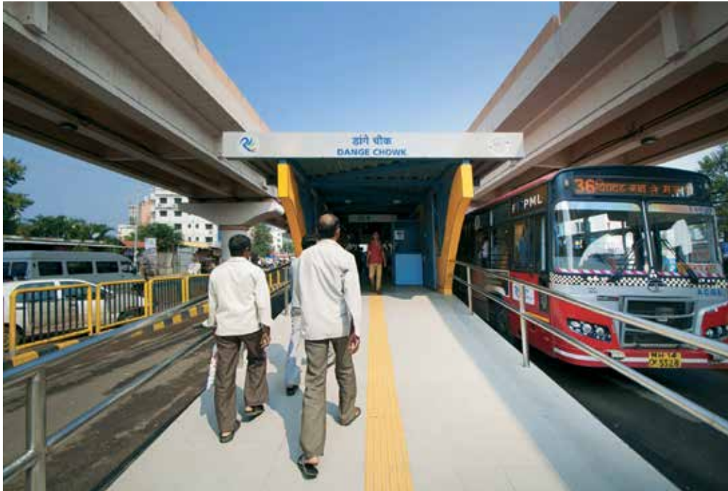
Photo 34: Station ramps enable all users to access the system comfortably (Rainbow BRT, Pimpri Chinchwad)
