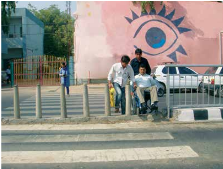
Photo 36: Inadequate spacing of bollards and level difference at crossings (Photo courtesy SAMARTHYAM)
