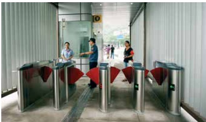
Photo 38: Flapgates and smart card readers control entry into stations and reduce fare evasion: Yichang BRT (left), Chengdu (right).
