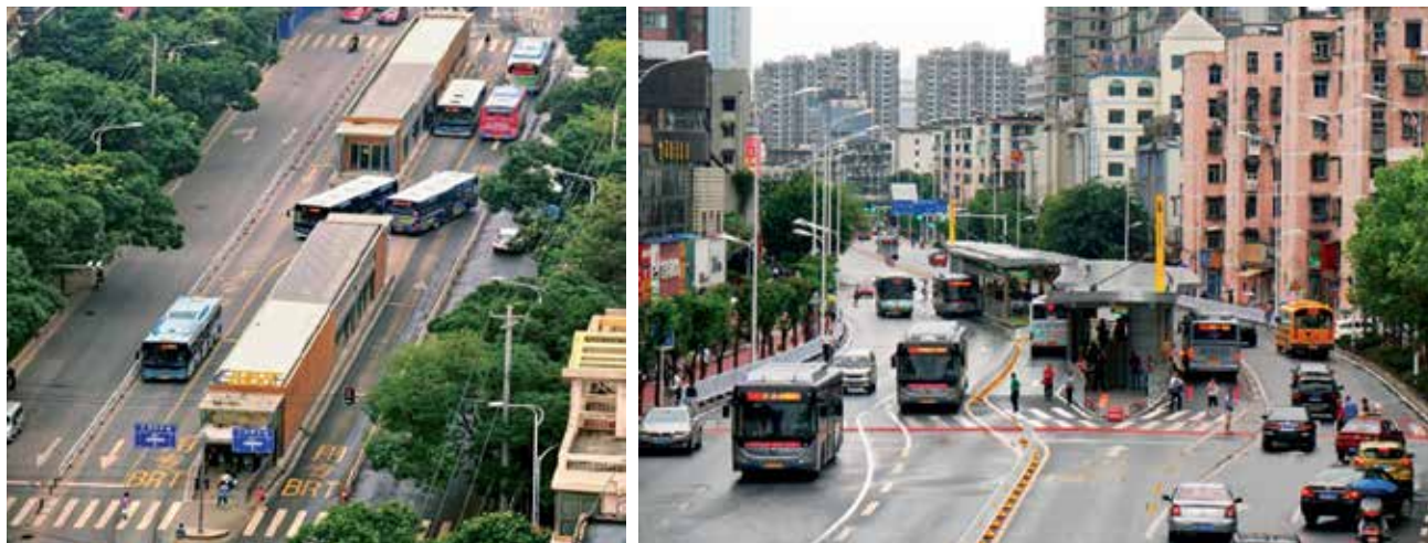
Photo 9: BRT stations with dual-side docking for buses traveling in a single direction in Lanzhou (left) and Yichang (right).
