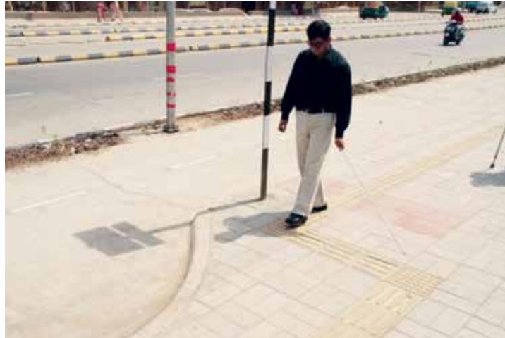
Photo 31: Tactile paving on footpath for persons with visual impairments (Photos courtesy: SAMARTHYAM)
