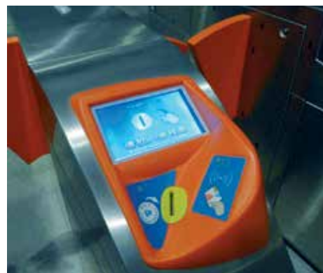
Photo 38: Flapgates and smart card readers control entry into stations and reduce fare evasion: Yichang BRT (left), Chengdu (right).
