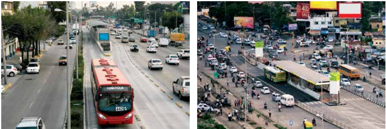
Photo 6: A single-lane BRT system like that in Mexico city (left) can handle volumes from 5,000 to 12,000 pphpd, depending on the type of vehicle used. With passing lanes at stations, a BRT system can carry up to 45,000 pphpd, the capacity of Bogotá's Transmilenio. iBus, Indore (right) has passing lanes at stations to help cater to future demand. (Photos courtesy ITDP and WRI India Sustainable Cities.)
