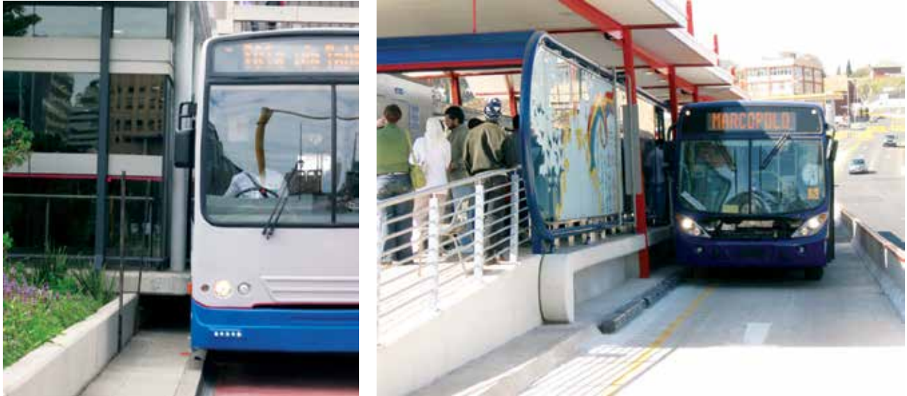
Photo 13: Kassel kerbs in Cape Town (left) and alignment markings in Johannesburg (right) help buses dock at BRT stations. (Photos courtesy UN-HABITAT)
