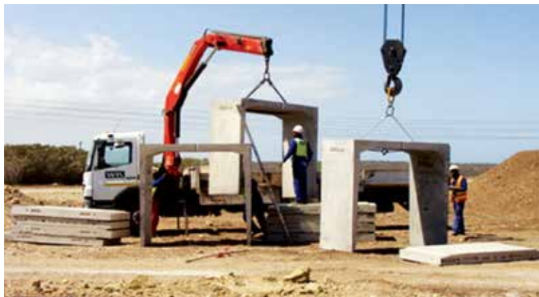
Fig. 13 Lifting and Placing of Box Segment
