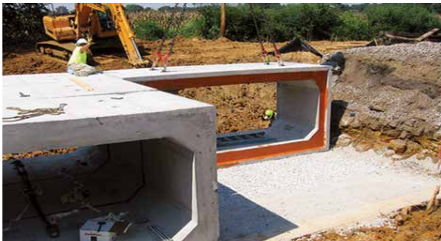
Fig. 14 Bedding Below Precast Concrete Segmental Box Cell
