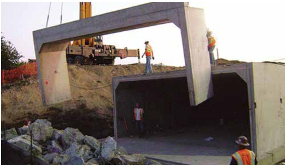
Fig. 15 Placing of Section of Box Culvert
