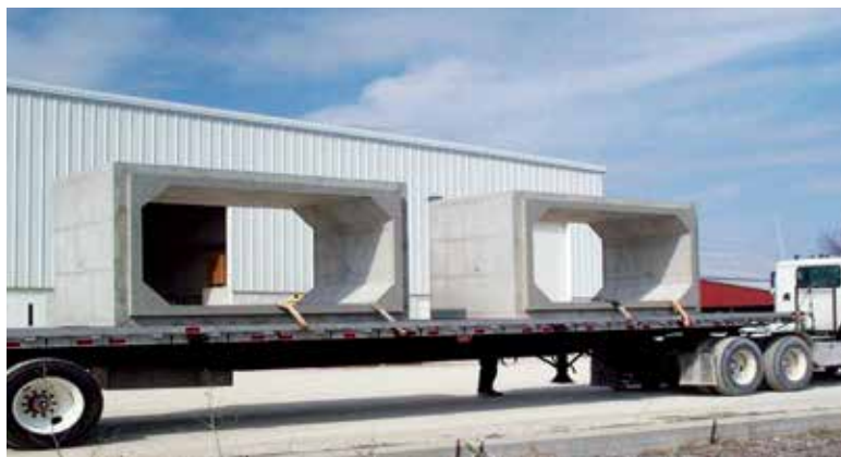
Fig. 11 Transportation of Sections of Box Culvert
