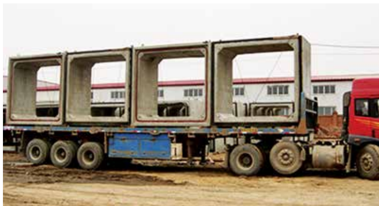
Fig 12 Transportation of Sections of Box Culvert
