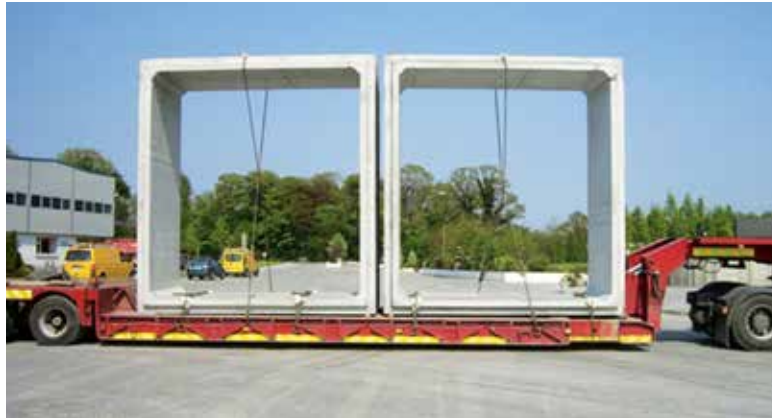
Fig. 10 Transportation of Sections of Box Culvert
