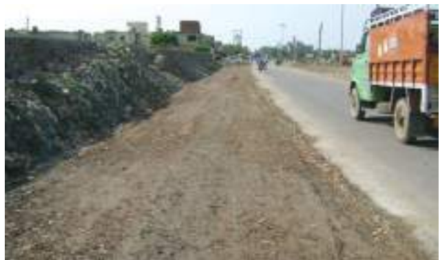
Photo 5 Cement Stabilised Base Course of C&D Waste Test Road
