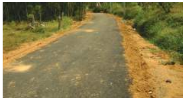
Photo 2 Another View of Rural Road Constructed Using C&D Waste
