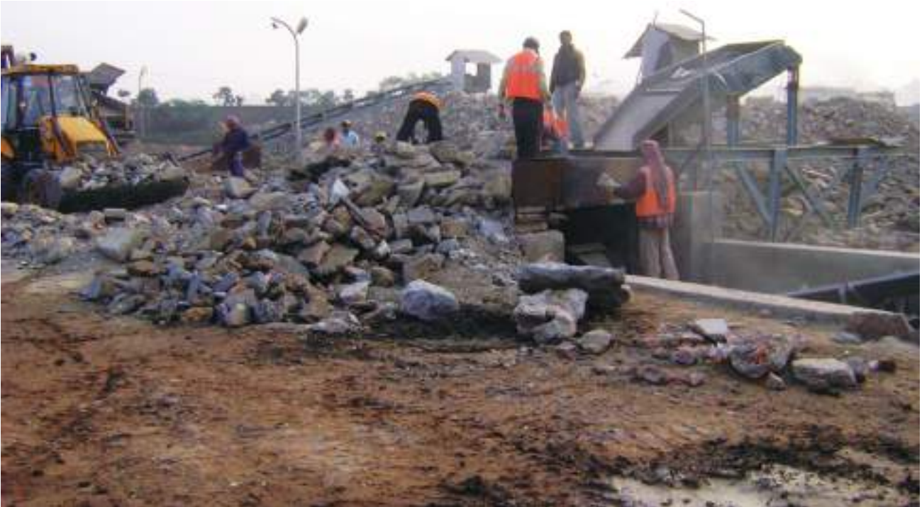
Photo 3 Dry Processing of C&D Waste
