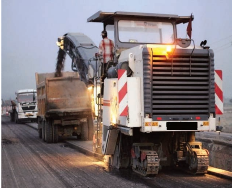
Photo 16. Milling the Bitumen Crust for FDR
