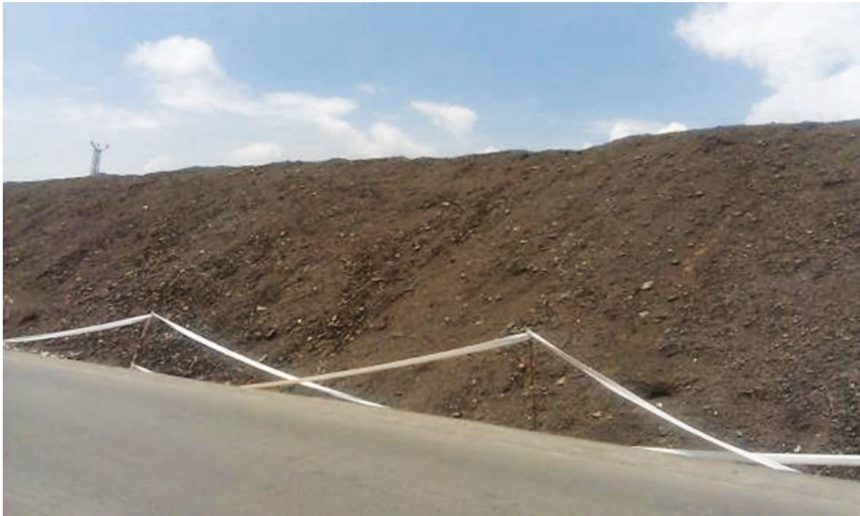
Milled Material stock piled after Milling
