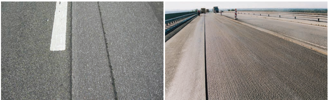
Photo 9: Good surface after milling
