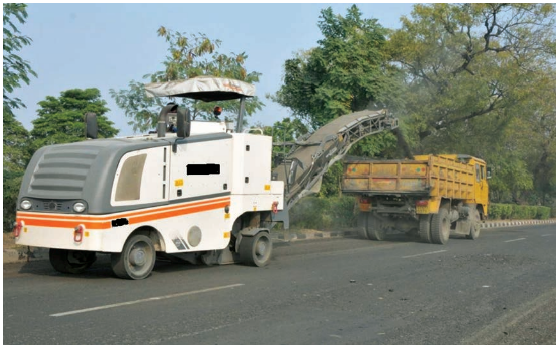
Photo 8. Milling in Operation
