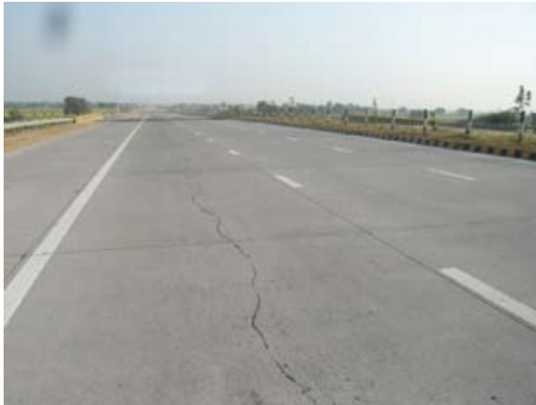
Photo 1 Longitudinal Cracks
