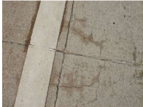
Photo 2 Corner Cracks
