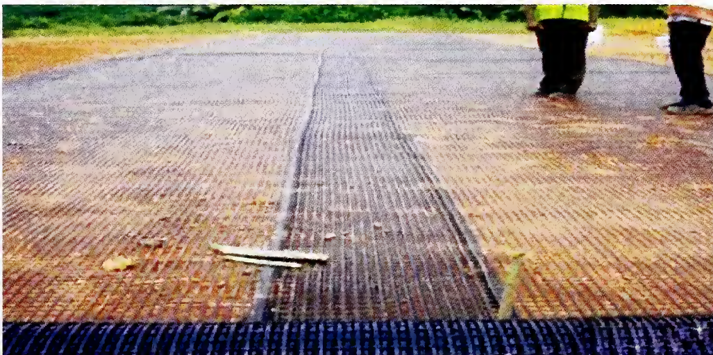
Fig. 17 : Installation of Woven Geogrids over Geotextile Separation Layer
