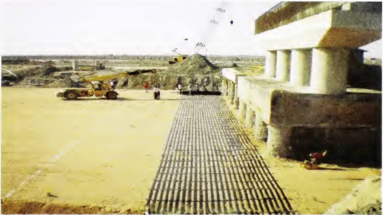
Fig. 28 : Installation of Bonded Geogrid, Mundra, Gujarat
