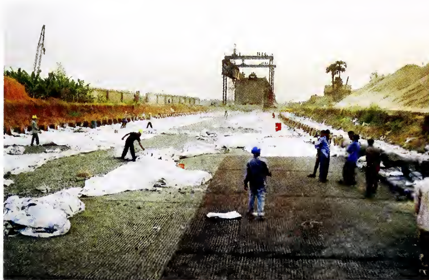
Fig. 23 : Construction of Basal Mattress at NH-5
