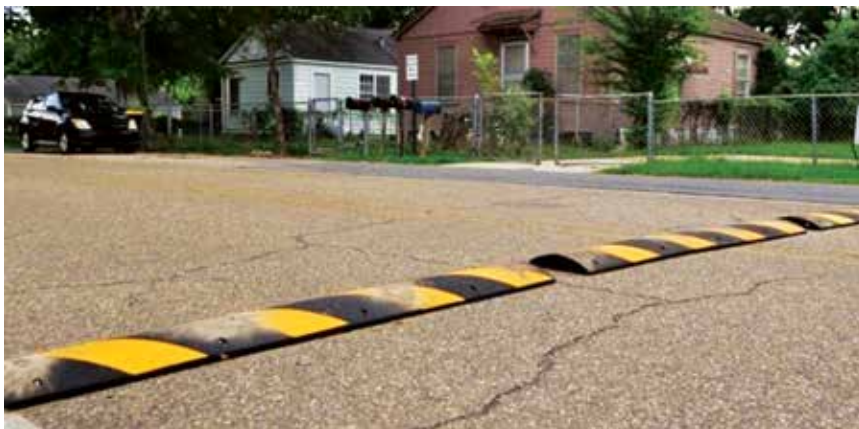
Fig. 3.5 Road Bump in Wide Residential Street (Gap in the Bump shown in fig. is a Traffic Hazard)
