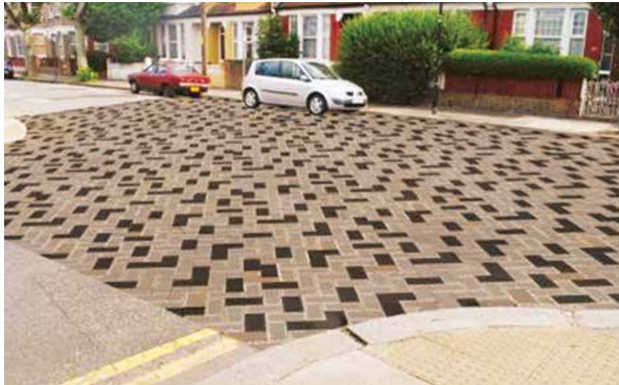
Fig. 2.12 Textured Paving over Raised Crossings
