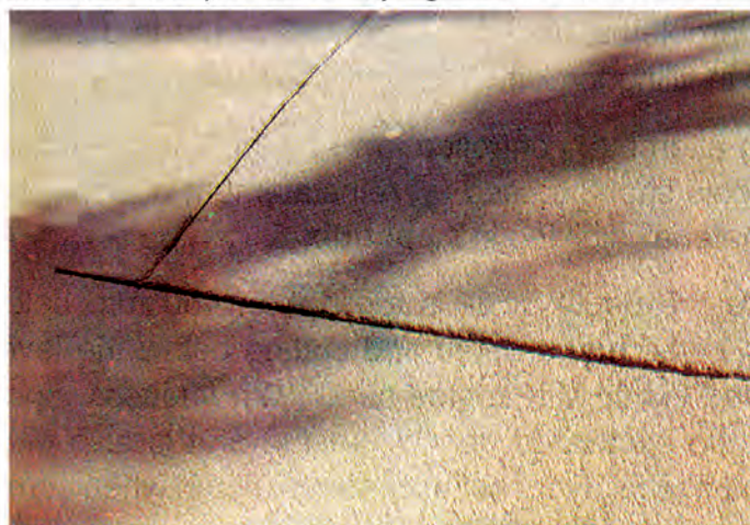
Photo-7 Sample of Poor Restoration of Surface Opened for Laying Cable
