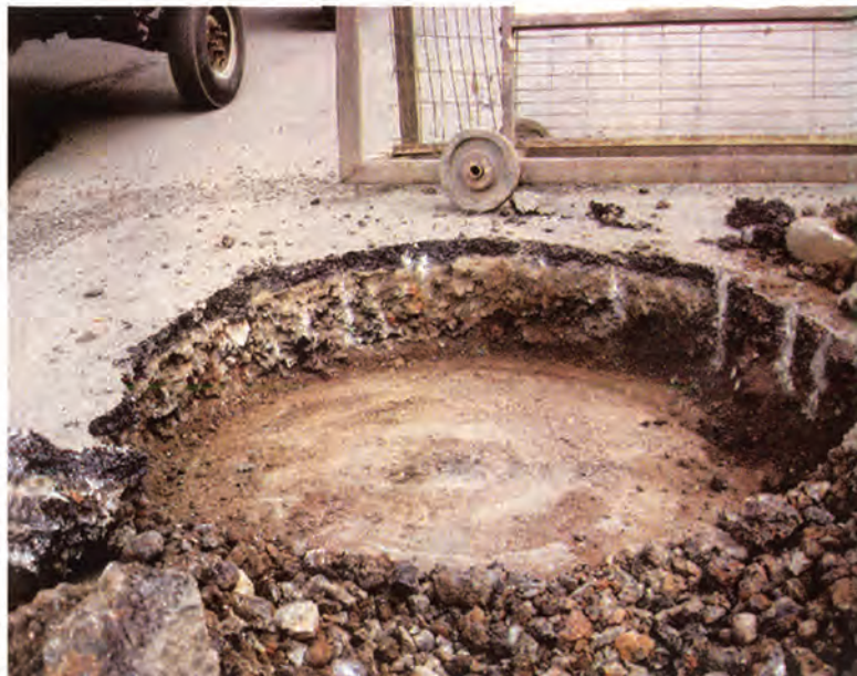
Photo-1 A Manhole Buried during Overlay Being Opened
