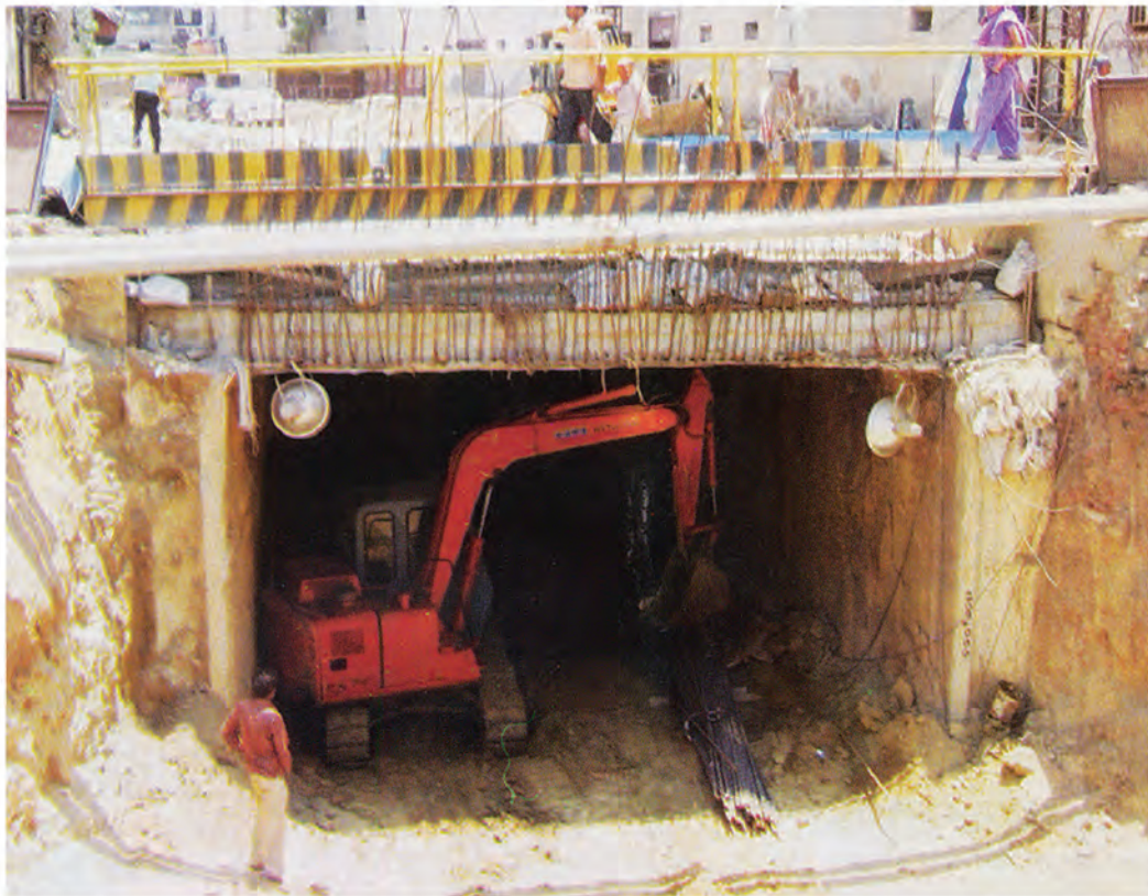
Photo-4 A Typical Multi Utility Service Tunnel under Construction – at Connaught Place, New Delhi
