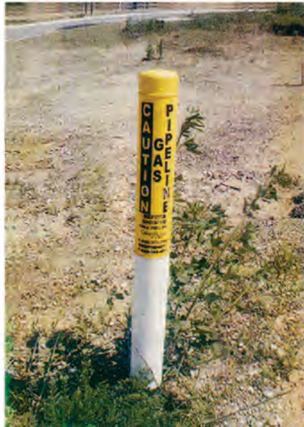
Photo-2 Sample Photo of Buried Gas Line Marked on the Ground
