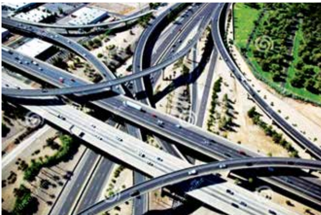
Fig. 3.9 Stack Interchange
