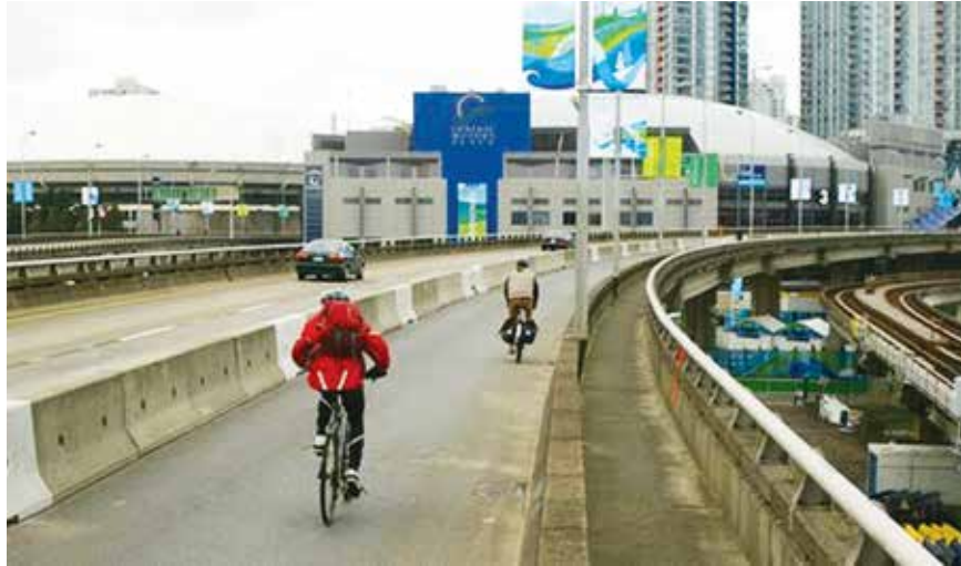
Fig. 9.4 Example for Dedicated Bicycle/Pedestrian Lanes Provided for Interchange at Vancouver, Canada
