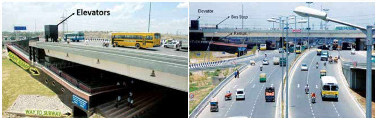
Fig. 10.1 Integration of Pedestrians at Mukarba Chowk Flyover using Elevators and Ramps
