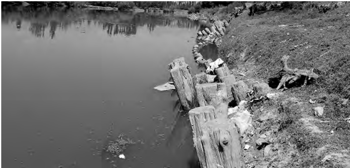
Fig. 6.10 Wooden piles over River Jhelum
