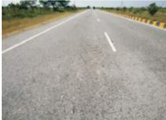
Photo 7.2.4 View of Dry and Hungry Surface
