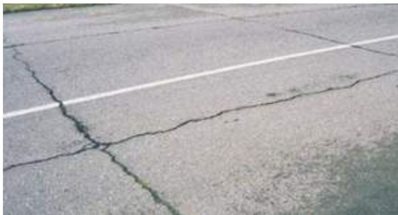
Photo 7.3.7 Reflection Cracking
