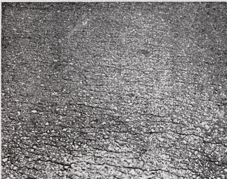
Photo 5. Hair-line cracks
