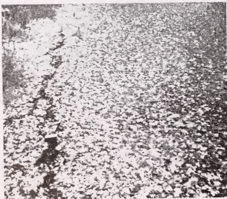
Photo 8. Edge crack
