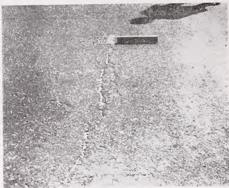
Photo 7. Longitudinal crack
