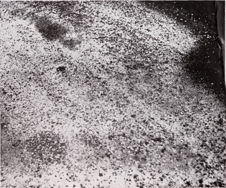
Photo 19. Loss of aggregate
