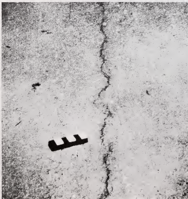
Photo 10. Reflection crack
