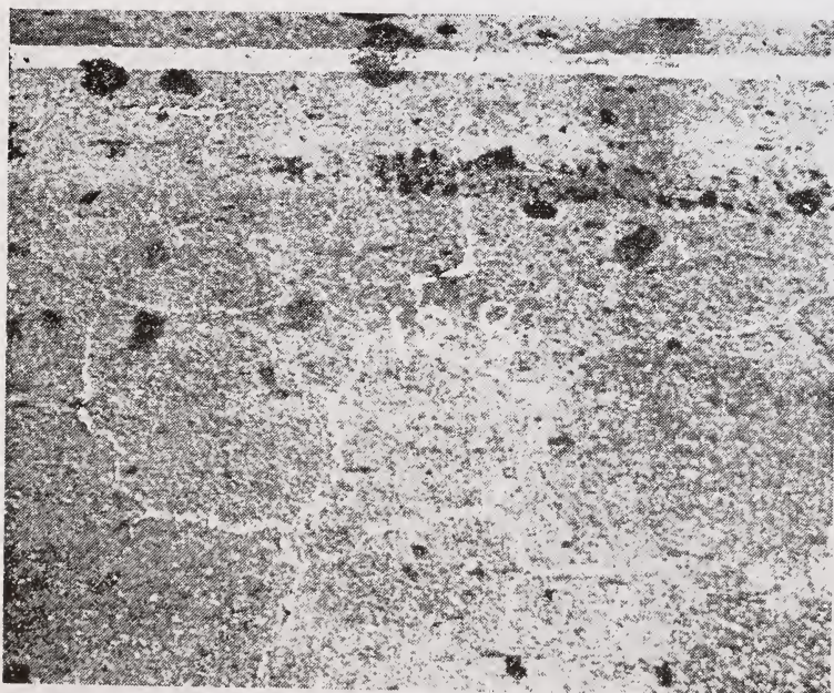
Photo 6. Alligator cracks
