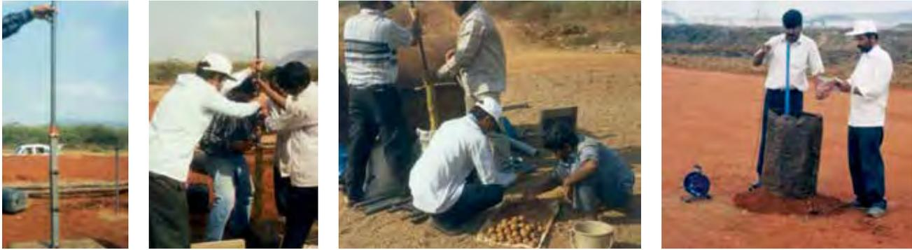
Ceramic Tip      Covering Tip      Bentonite Pellets      Monitoring Pore water
