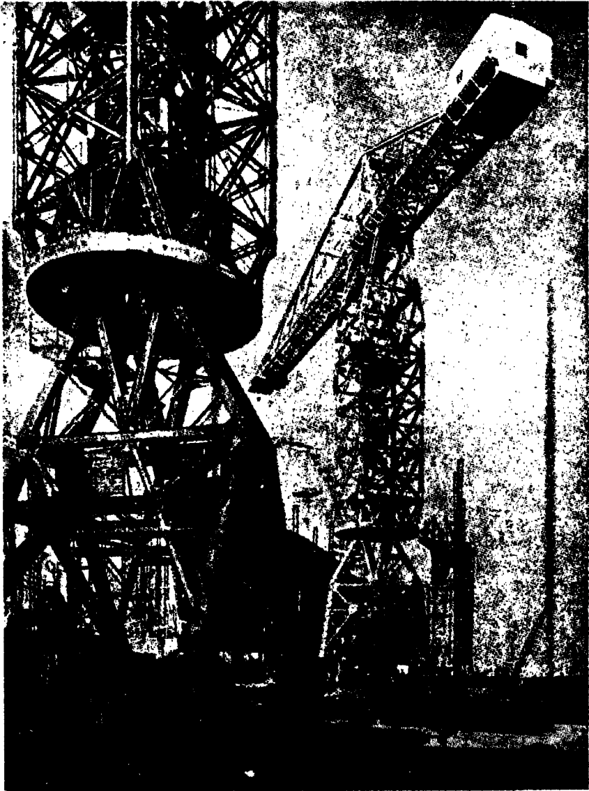
FIG. 4 GOLIATH CRANE (GENERAL VIEW)
